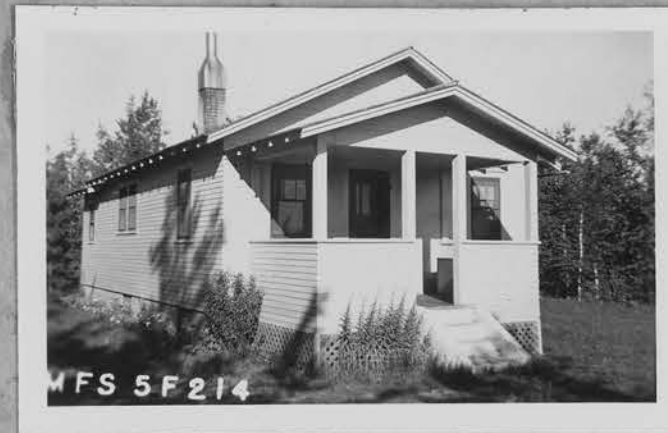
No. 38 Subject LOOKOUT CABIN 5+214 Negative ----- Print ----- Slide ----- Cut Taken by ----- Place BEMIDJI Date -----
