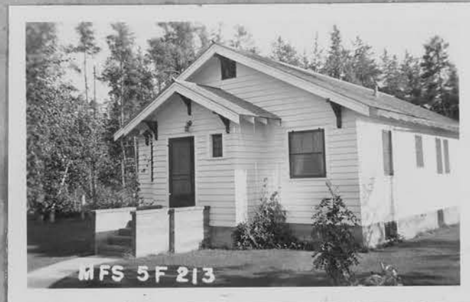
No. 37 Subject RESIDENCE CABIN 5+213 Negative ----- Print ----- Slide ----- Cut Taken by ----- Place BEMIDJI Date -----
