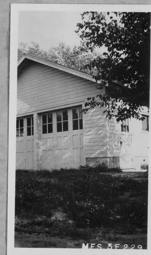
No. 358 Subject WAREHOUSE
