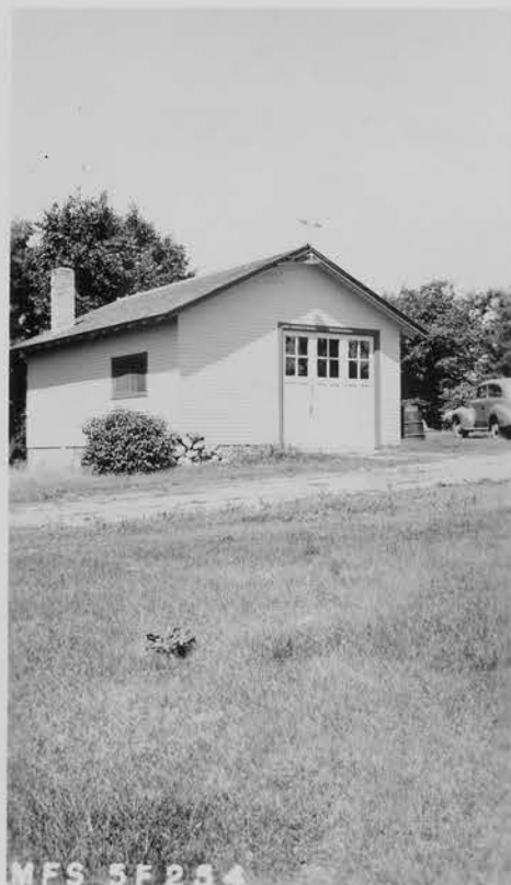
No. 147 Subject WAREHOUSE
