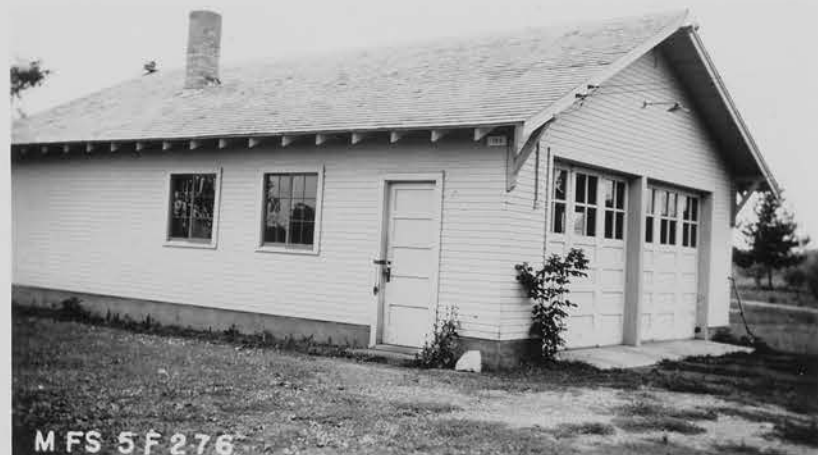
No. 154 Subject RANGER STATION 5f276 Negative FAS 10 WHSE Print Slide Cut Taken by Place ONAMIA Date
