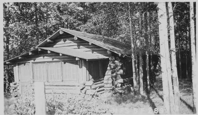
No. 113 Subject OFFICE-BUNKHOUSE 5F289 Negative ..... Print Taken by ..... ..... Slide Place FINLAND ..... Cut Date .....
