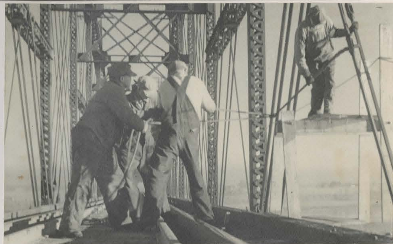
38-316 TIGHTENING EYEBARS
