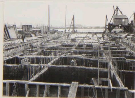
40-33-IN THE EMPTY GRAVING DOCK 40-29 A NEARLY COMPLETED PONTON
