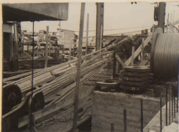
40-43 THE EYEBARS ON THE LEFT EACH ANCHOR TWO STRANDS OR 664 WIRES, EACH CABLE WILL HAVE 6308 WIRES...
