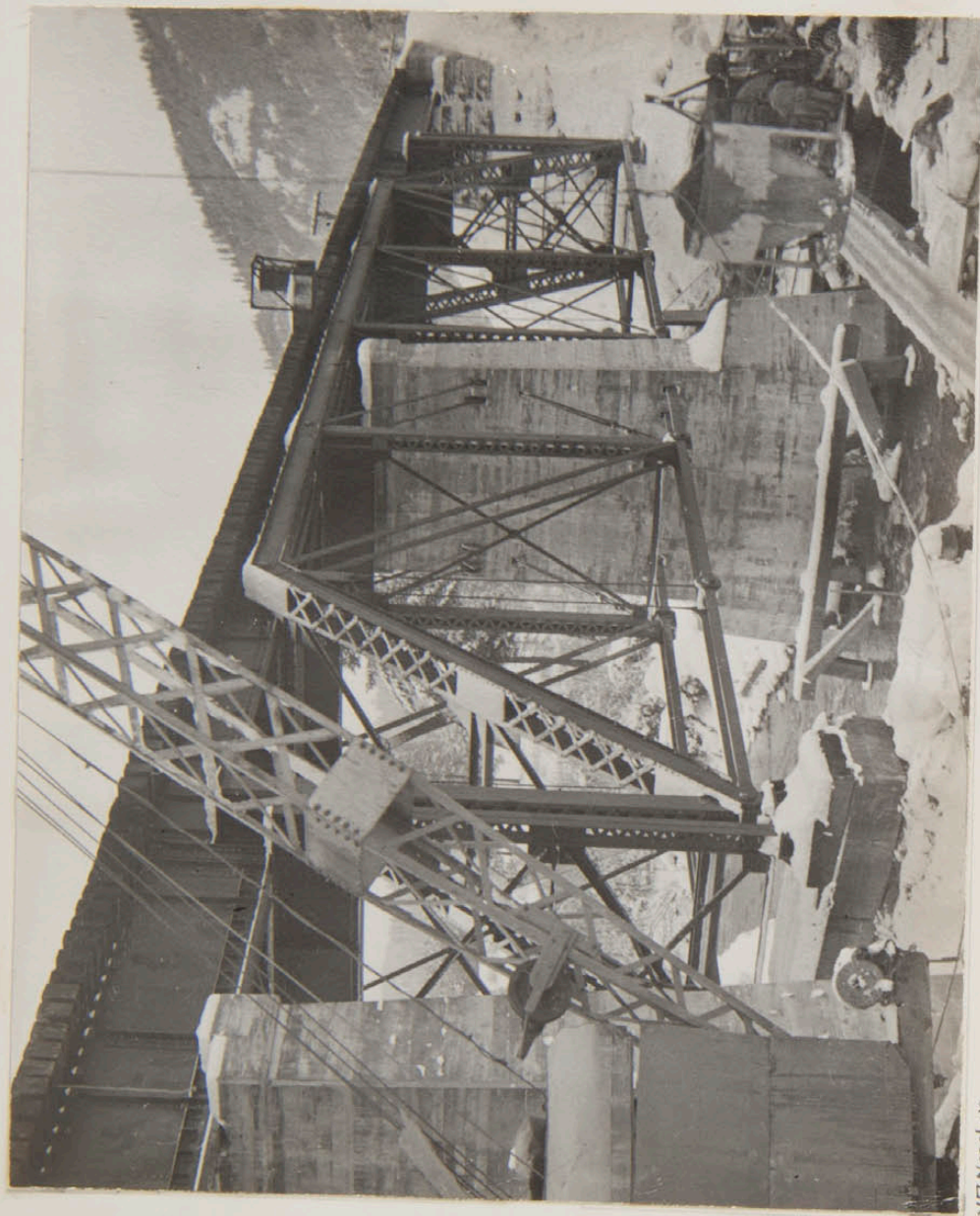
ADDING A PIER AT TROUT CREEK
