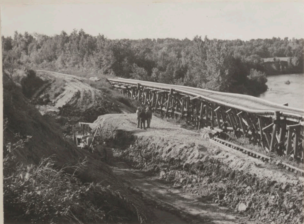
SLIDE-OUT OF NEW FILL NEAR RED LAKE FALLS
