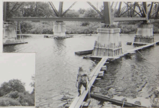
Intrusion-Prepakt Repairs at Valley City Viaduct.....
