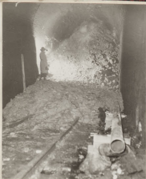
WEST FACE OF CAVE-IN -- SHOWING JACKED PIPE
