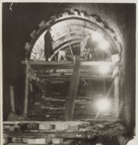
RAIL ARCHES AND LAGGING -- -- -- WEST FACE
