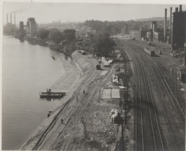
FILLING FOR THE NEW RIVER ROAD EXTENSION
