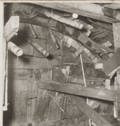
GROUT PIPES DRIVEN INTO EAST FACE OF SLIDE.
