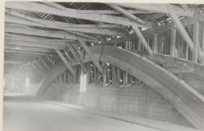
55V-93 Framework of Covered Bridge at Bath, N.H.
