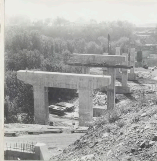
60-193 Most of the piers are nearly complete
