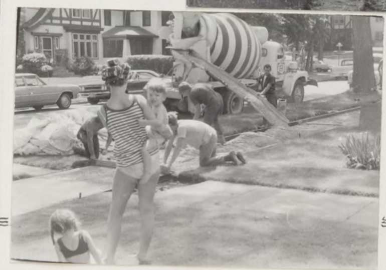
69-94C- Pouring and finishing the five-foot sidewalk- and some kibitzers.
