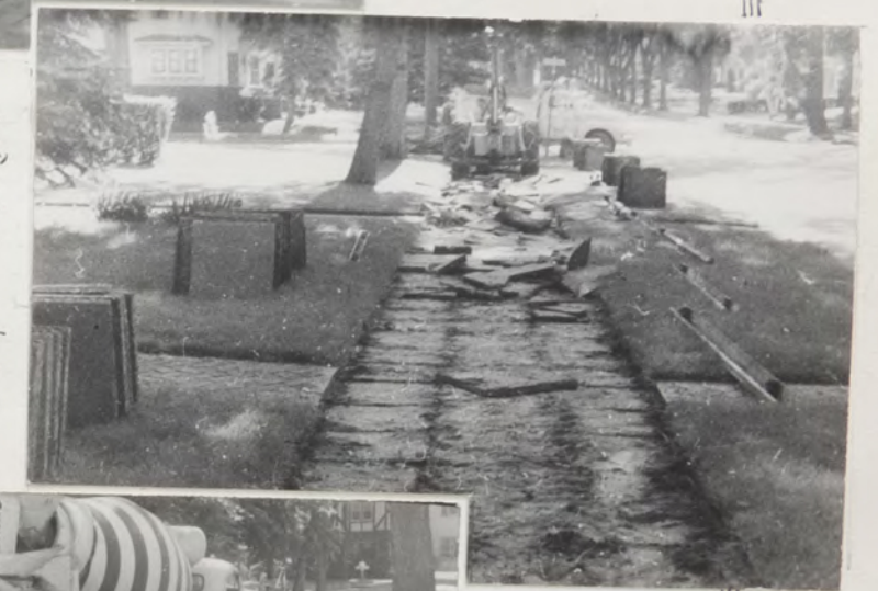
69-94B- East from our front brick walk- the ready-mix truck has a long trough to deliver the concrete to the new walk.
