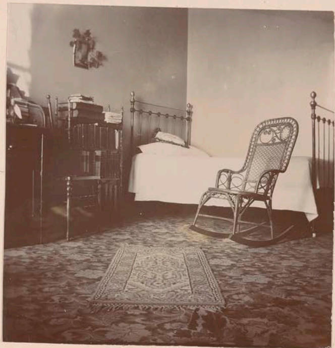
House Physicians Room (17)
