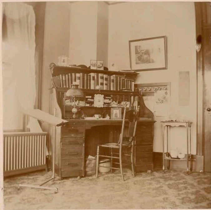
House Physicians Room (3)
