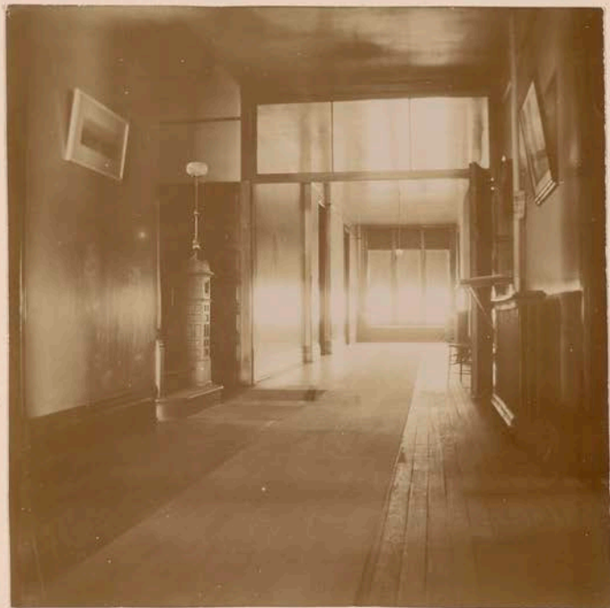
Corridor (first floor)
