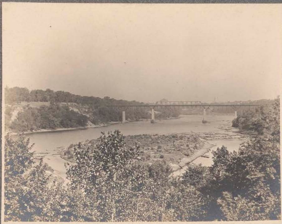
High bridge, St. Paul
