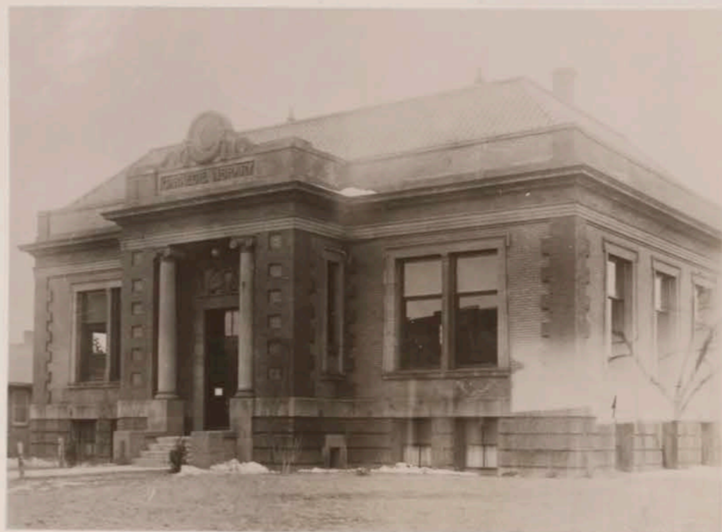
Carnegie Library, Hibbing, Minn.
