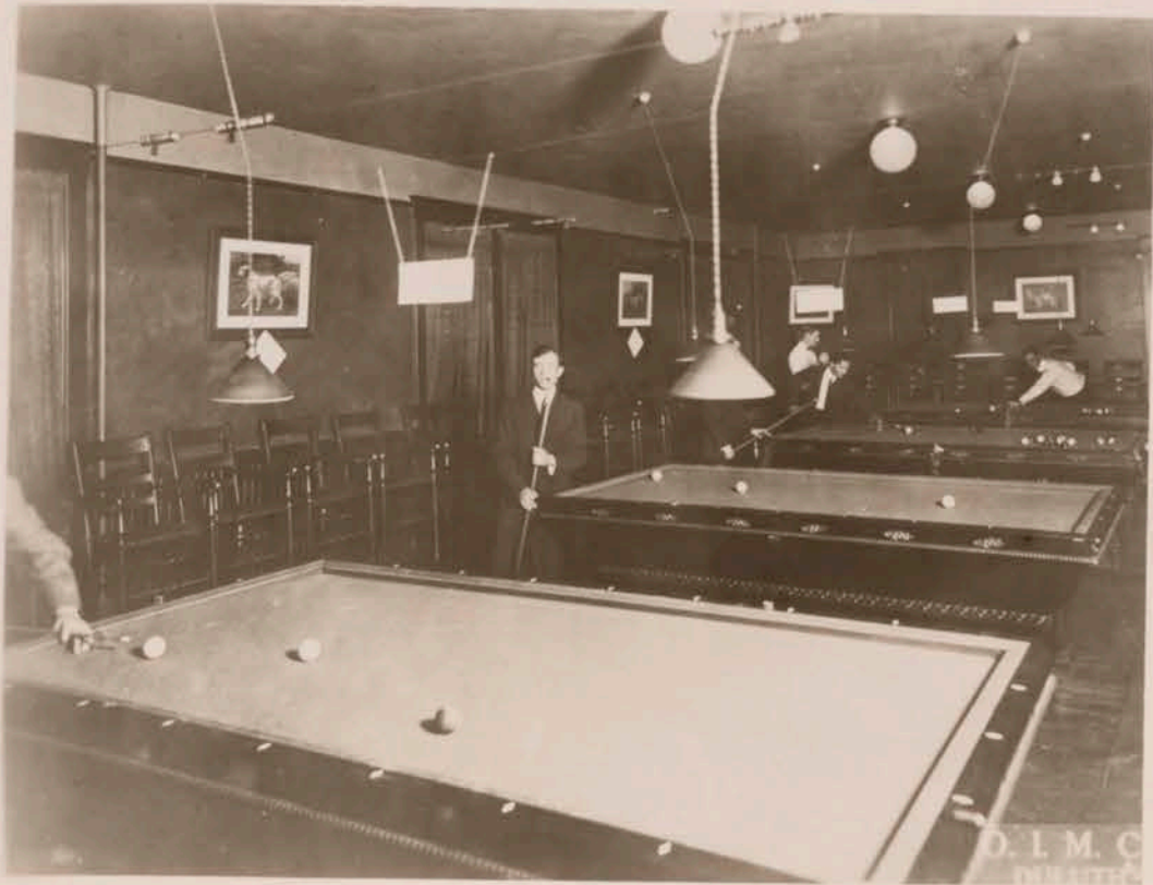
Billiard Room, Hibbing Club House
