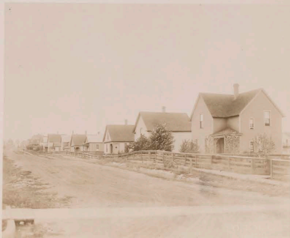
Mining Location, Adams District, showing workingmens houses.
