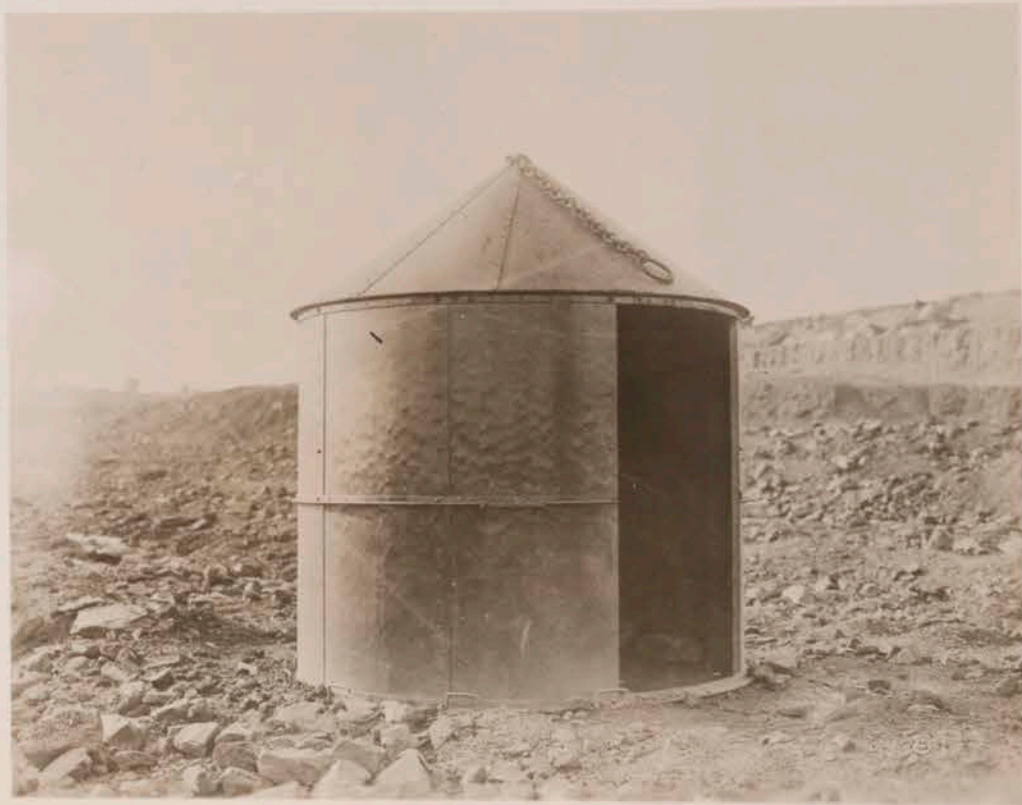
Shelter from blasting in pit.
