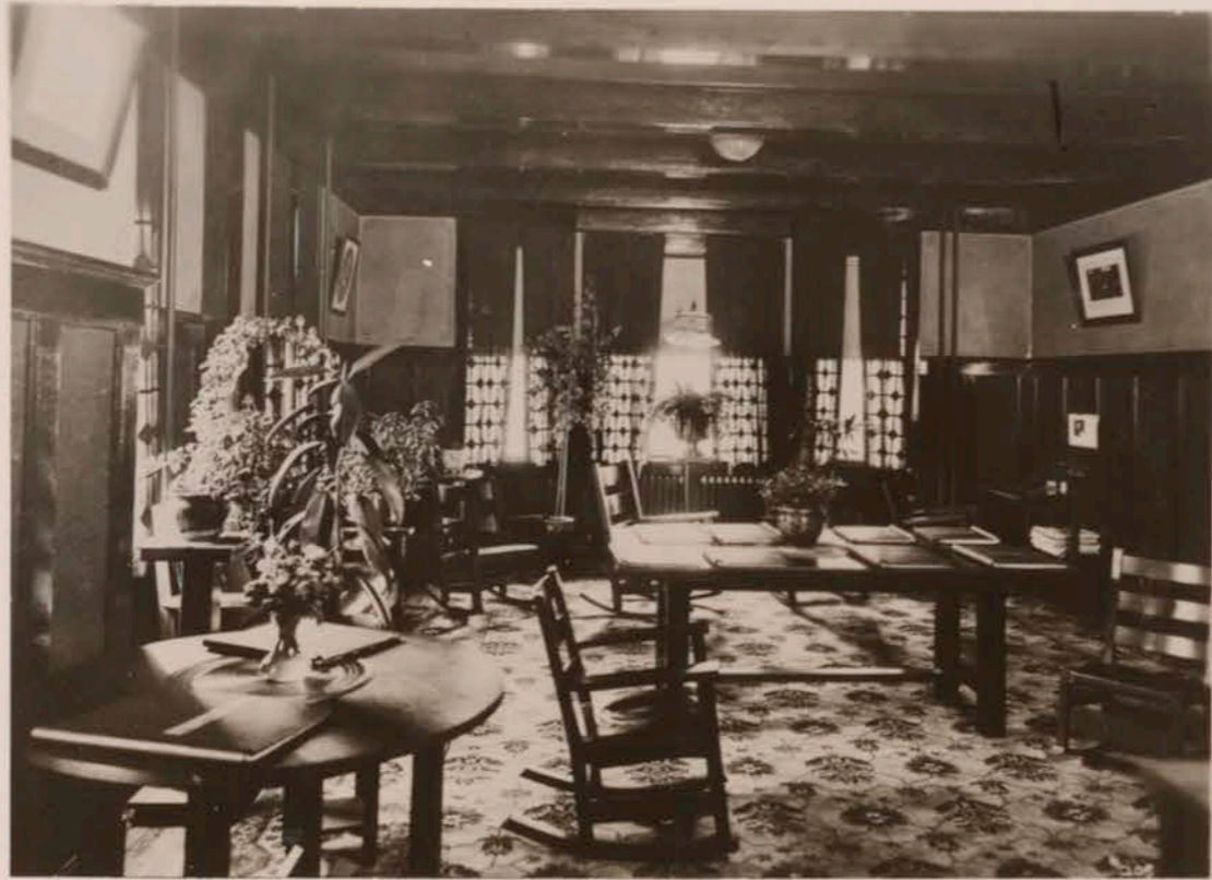
Rest room, Virginia Dist. Club house. Virginia District Headquarters.
