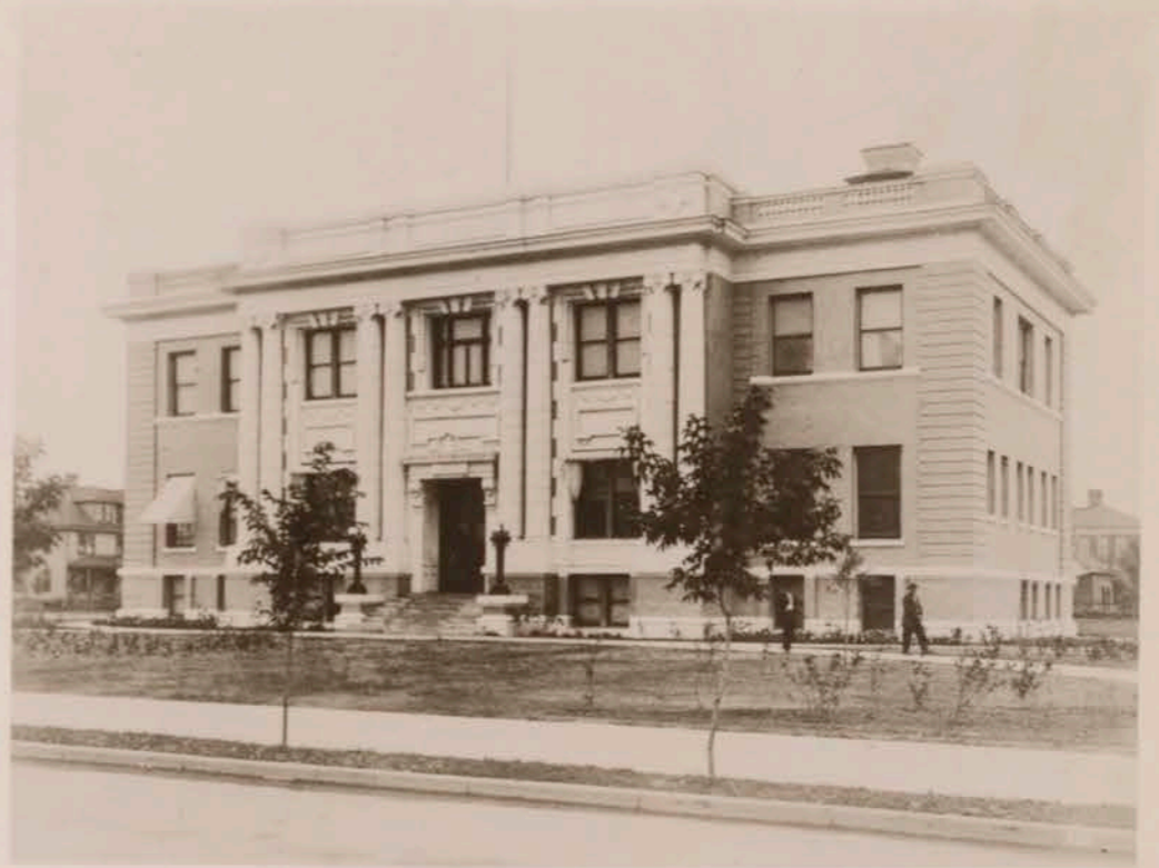
St. Louis Co. District Court House, Virginia Minn.
