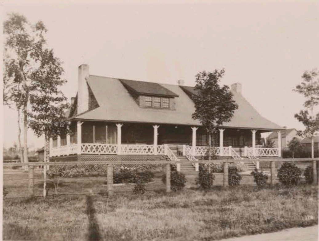
Residence of Asst. Gen'l. Superintendent Canisteo District, Coleraine, Minn.
