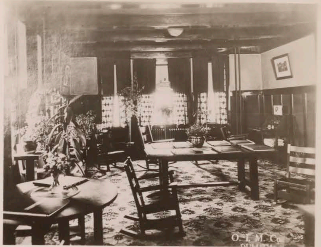
Rest Room, Virginia District, Club House
