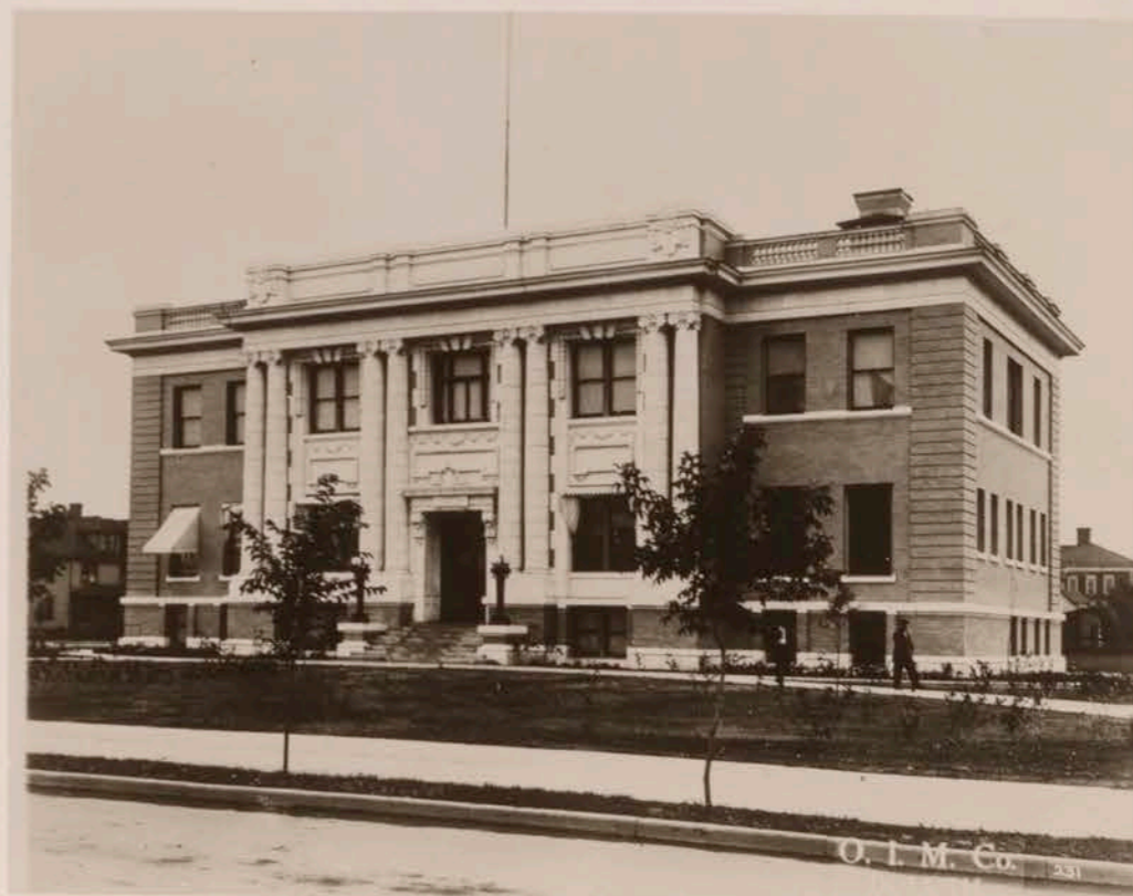
St. Louis Co. District Court House, Virginia, Minn.
