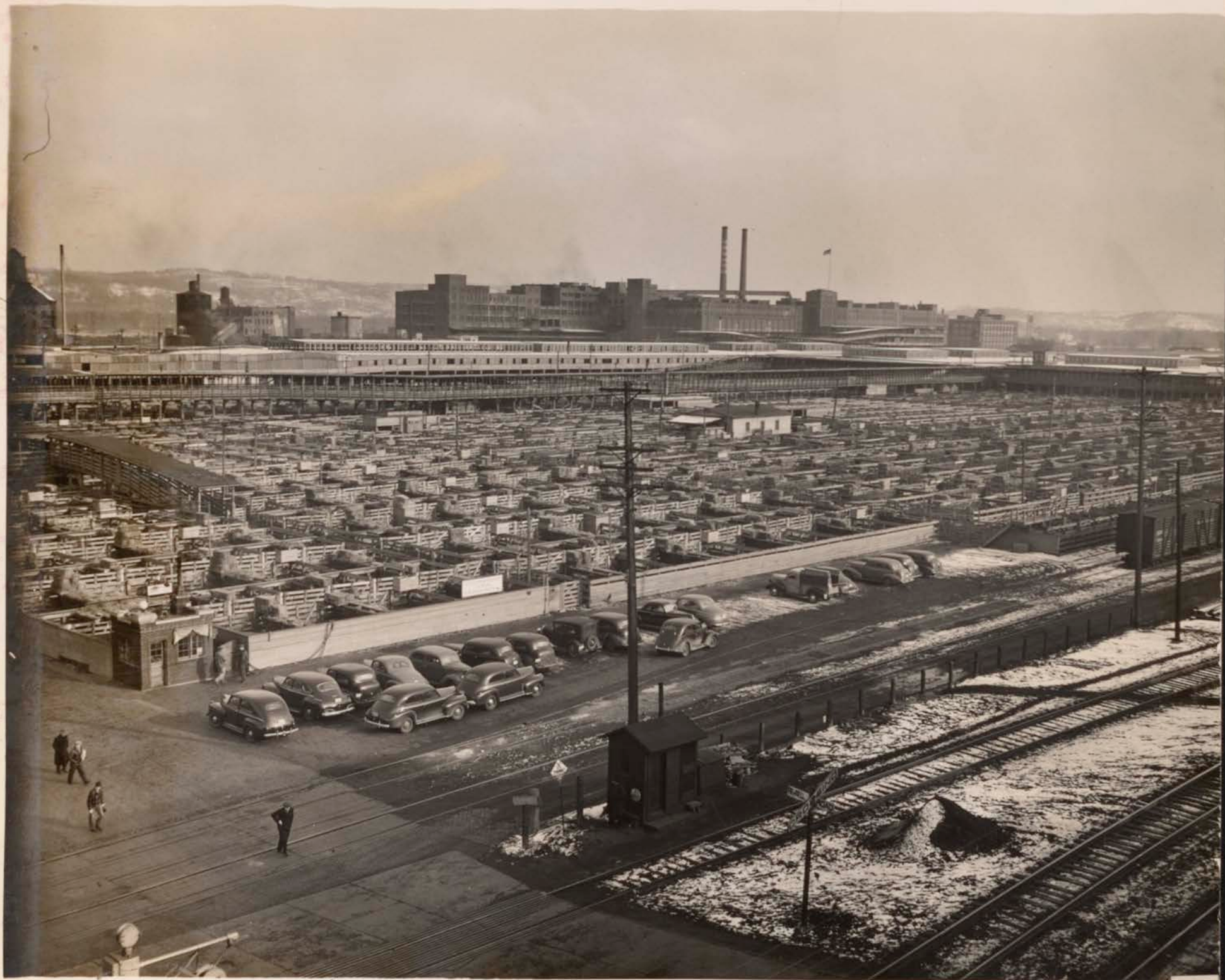
GENERAL VIEW OF YARDS
