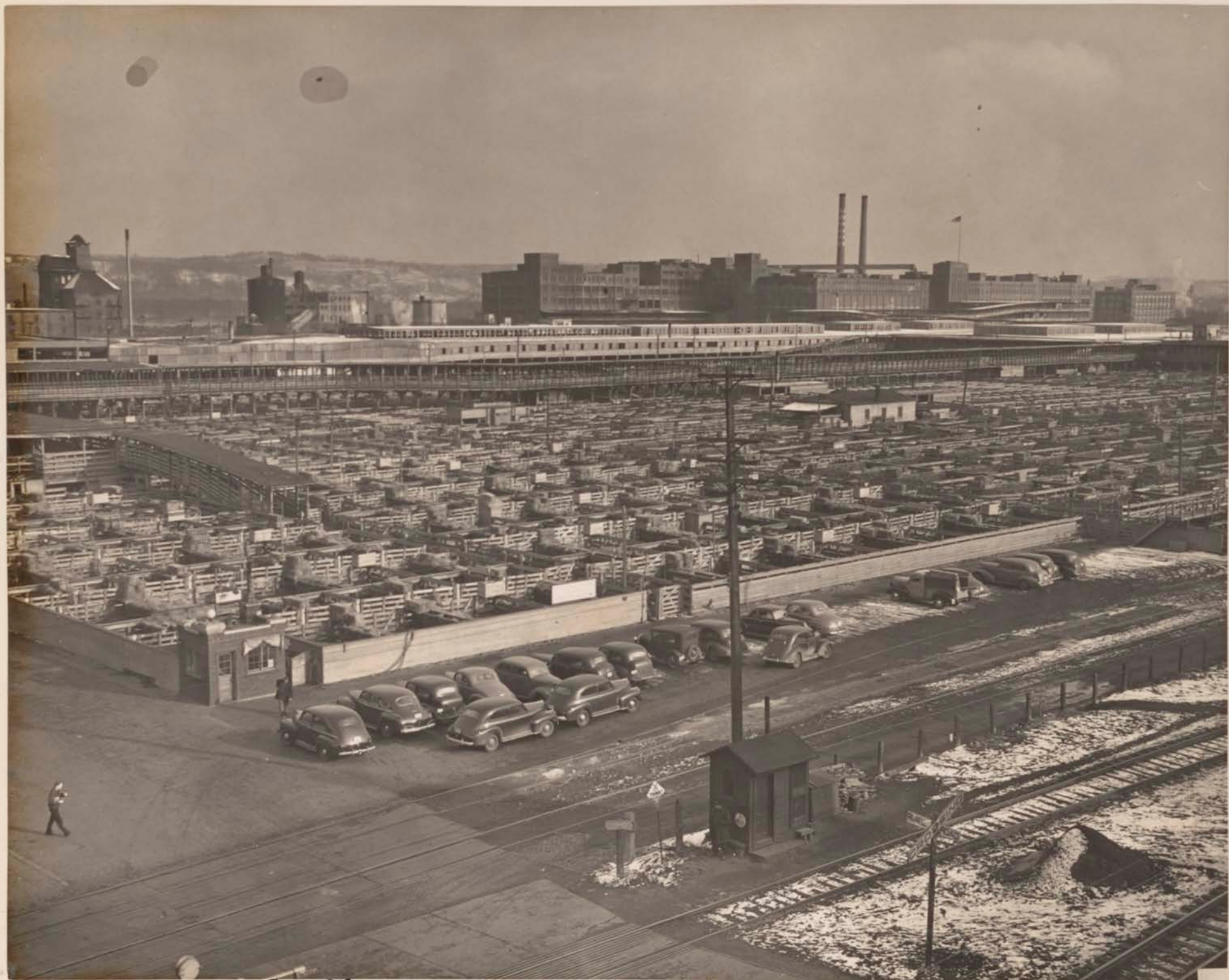
GENERAL VIEW OF YARDS
