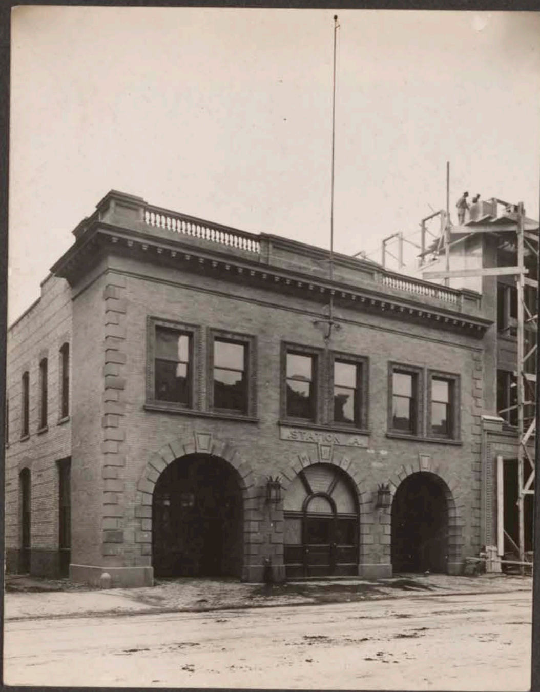
Fire Dept. Building 4th No., near Hennepin Built in 1902
