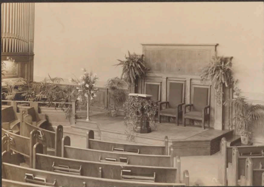
Remodeled & Refinished Interior of First Unitarian Church - 1912
