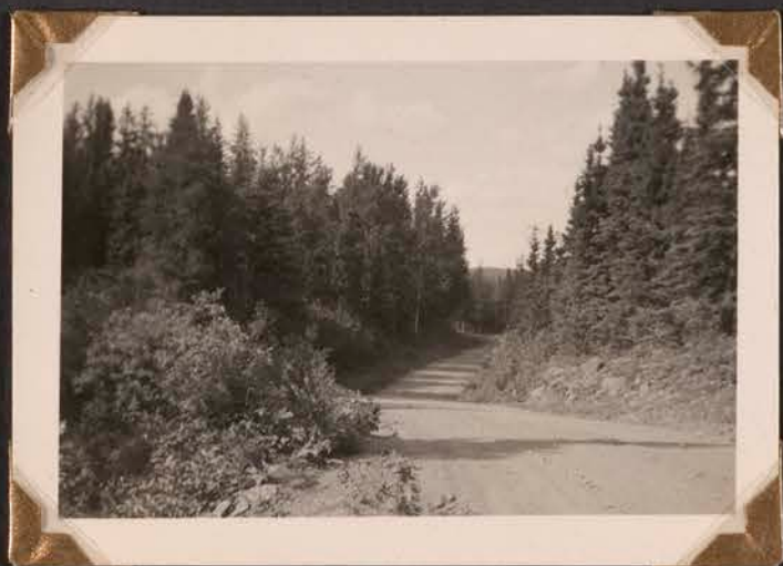
Southwestern entrance into CCC Co 712.
