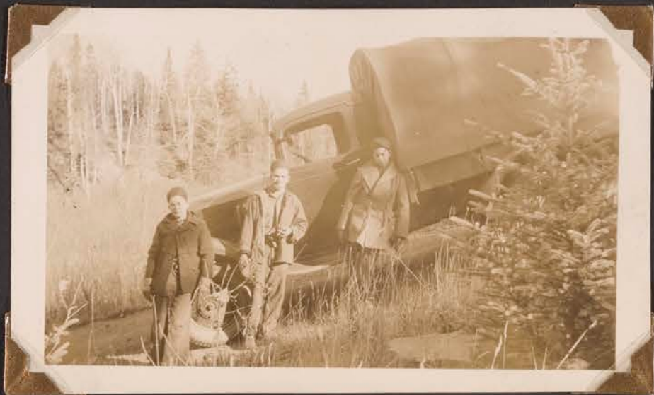
Ken Nelson Paul Mieimie Hugh Mullen and the Army Canvay enroute to Seagull Camp for some dismantling work.
