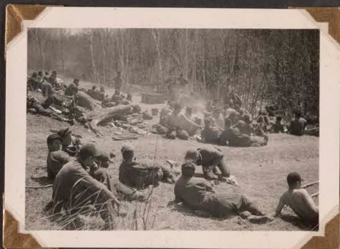
A job that the boys cheerfully looked to such as Partially broken backs twisted joints a hot blistering sun and all the vermin & bugs in the states
