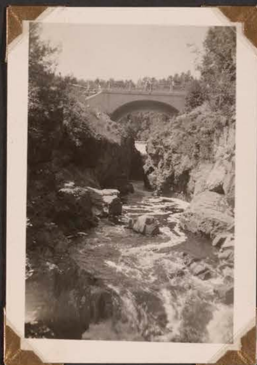
U.S. Highway No 61 where it crosses the Temperance River.
