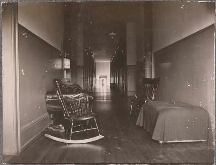
Main Hall 2 nd floor Sunward
