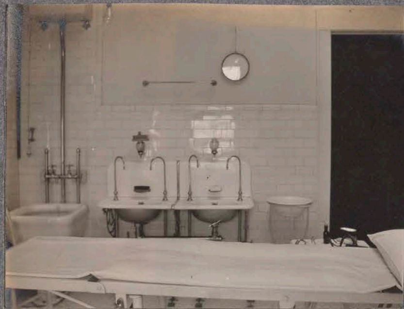
Operating Room 3rd floor M.S.F.H.
