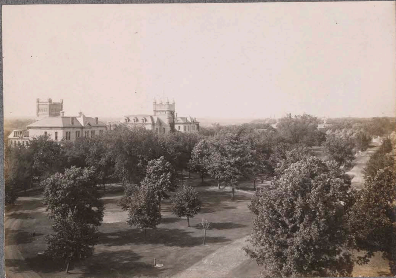
T.M. Campus from Sunny side Tower
