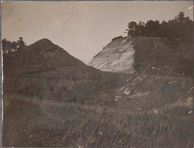
Rock Island Cut M.S.F.M.
