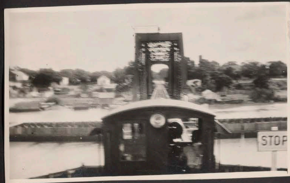
Q. P. bridge across Altamaha river at Marien, Ga 8-4-14
