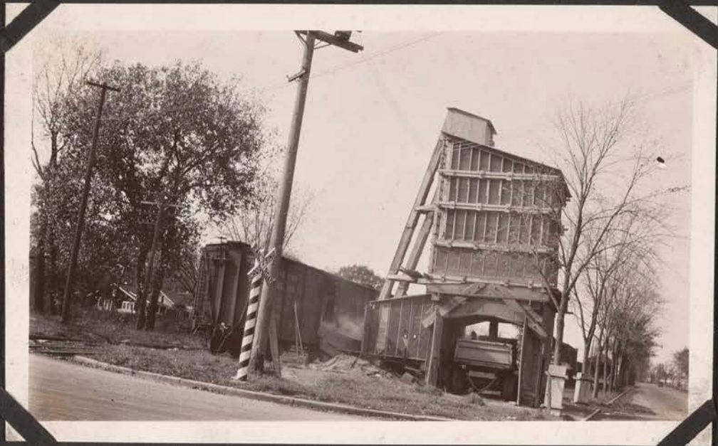
Bin for Handling Bulk Cement from Box Car to Truck.
