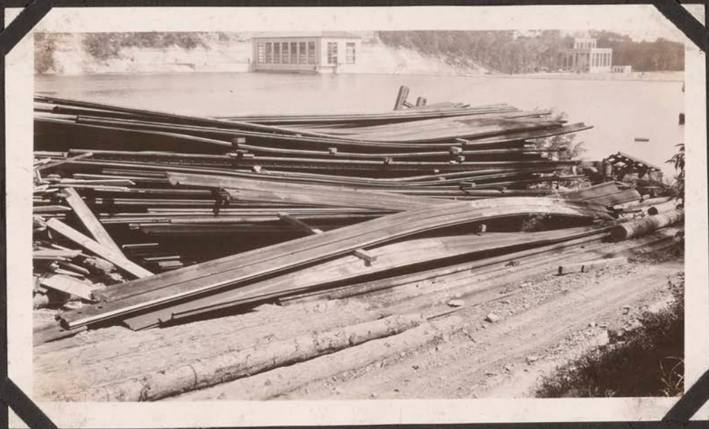
50ft. Sheet Piling pulled from Cofferdam.
