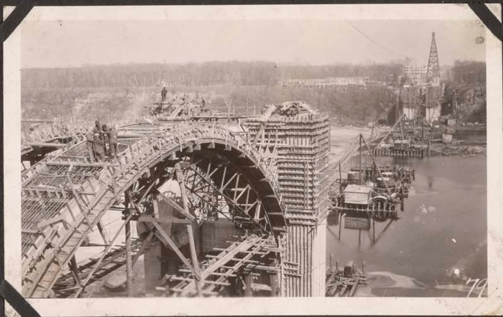
Progress View, Looking East Mar. 27, 1926.
