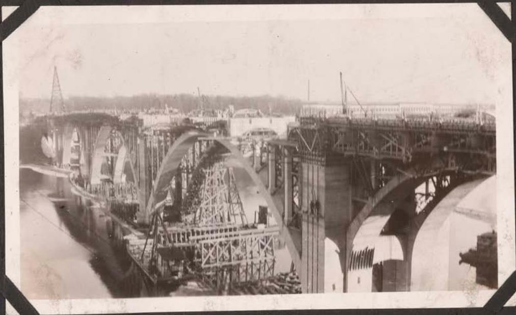
Progress View, Looking East, Oct. 27, 1926.
