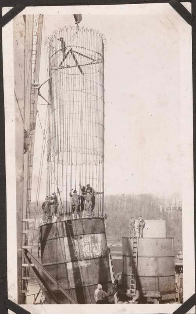
Placing Caisson Reinforcing Pier 9
