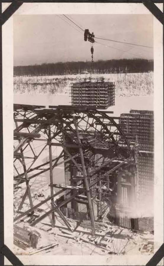
Placing Sectional Built Forms
