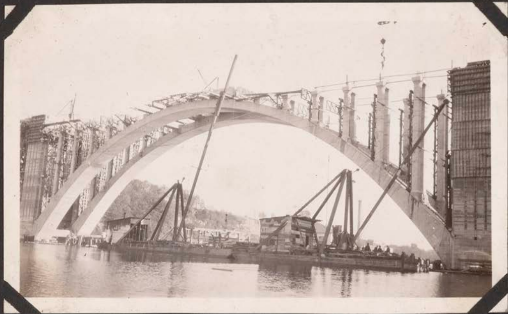
Northwest View of Ribs and Columns Span 8
