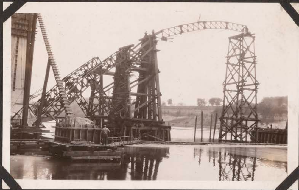
Erecting Arch Centering May 12, 1926.
