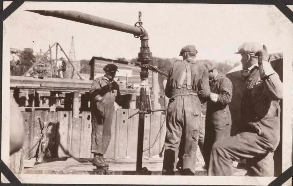
Sinking Caisson by Jetting
