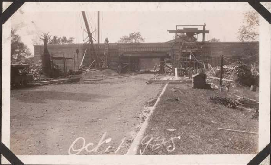
Godfrey Road Viaduct
