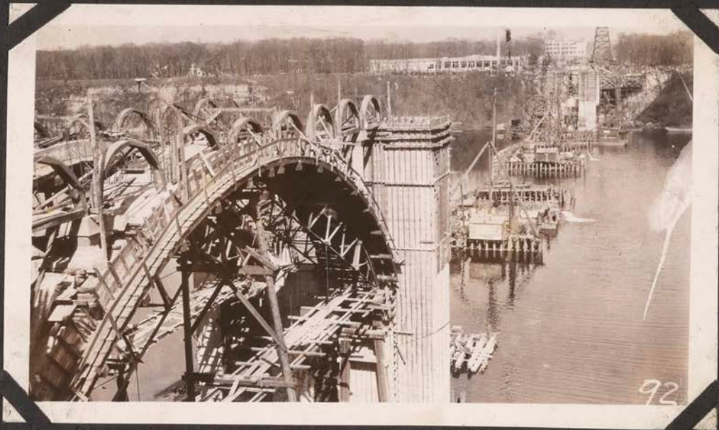
Progress View, Looking East Apr. 30, 1926.
