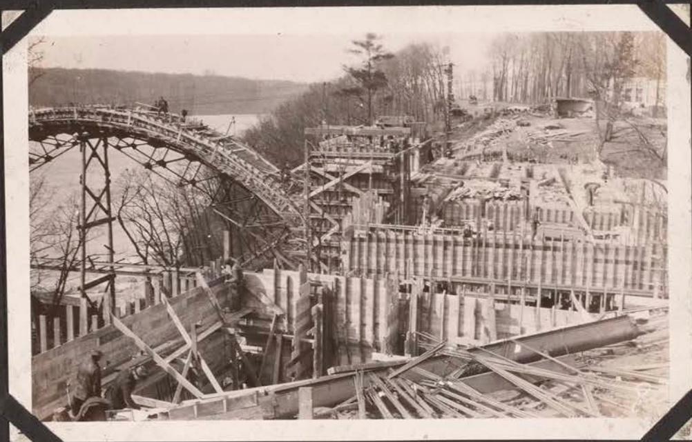
Building Forms For Under-Crossing Apr. 2, 1926.
