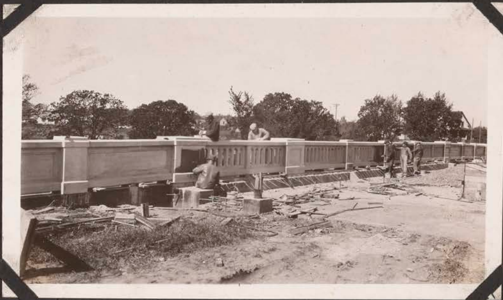
Godfrey Road Viaduct Rubbing Concrete Railing.
