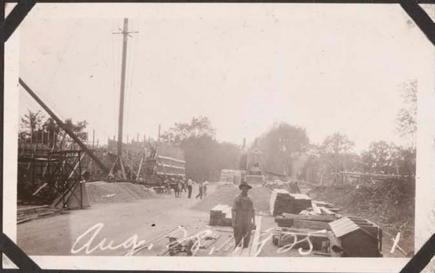
Godfrey Road Viaduct
