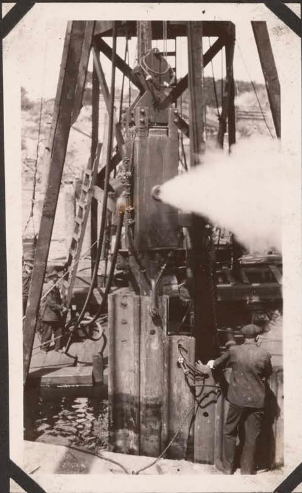
Pulling Sheet Piling with Steam Hammer Inverted.
