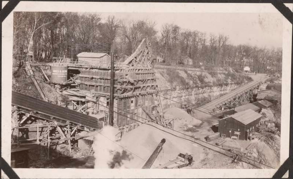
Mixing Plant and Shop Buildings 10-27-'26.
