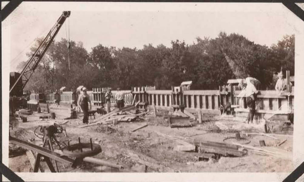
Godfrey Road Viaduct Building Forms for Railing.
