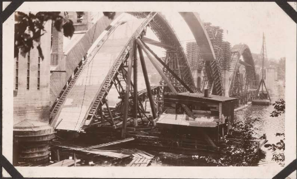
Removing Arch Centering
