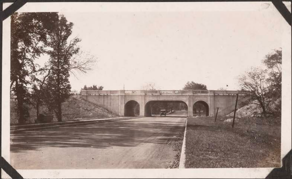
East Elevation of Godfrey Road Viaduct Sept. 25, 1926.
