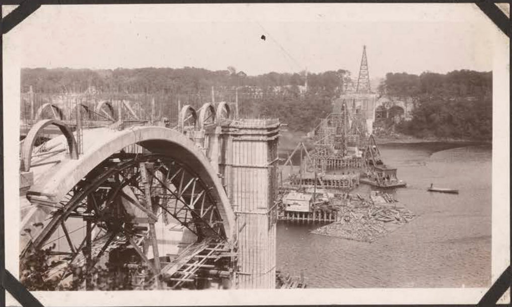
Progress View, Looking East May 28, 1926.
