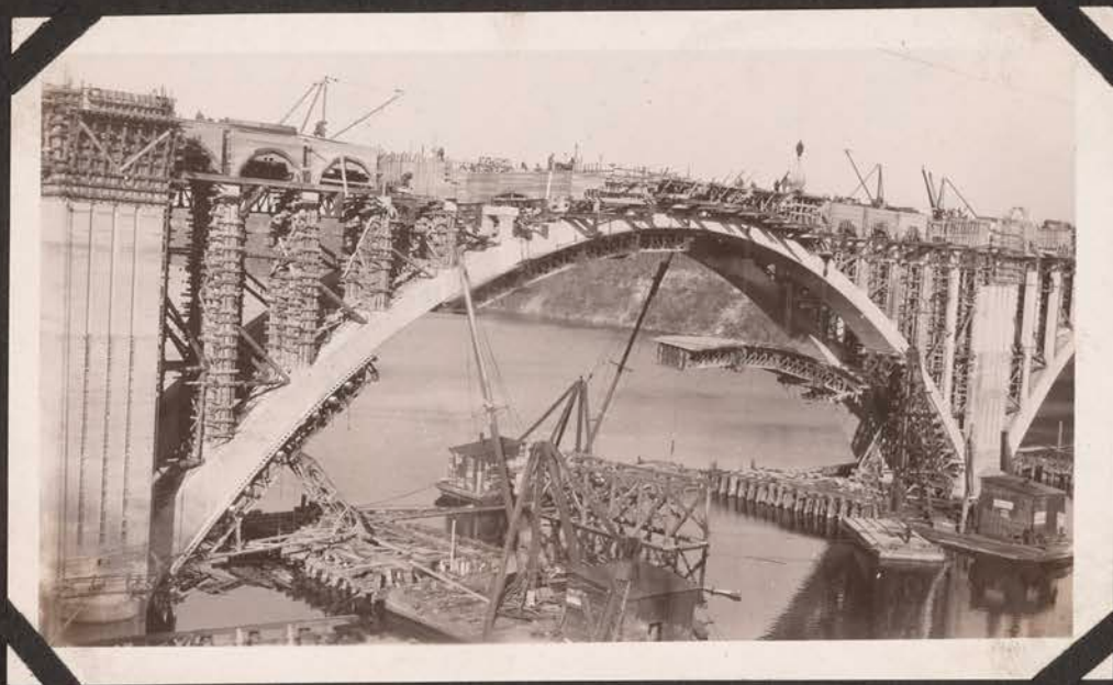
Lowering Steel Centering S. Rib Span 9.
