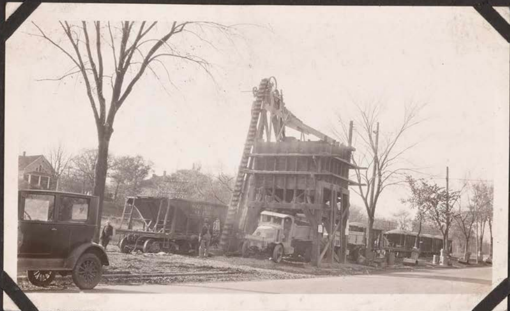
Unloading Crushed Rock from Cars.
