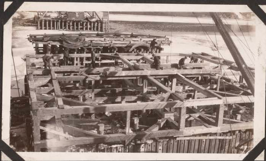
Cofferdam framing, Pier 9, Feb. 26, 1926.
