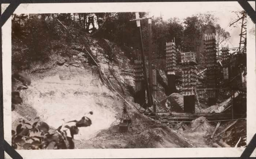
East Approach Oct. 1, 1925. Excavating for Pier 6.
