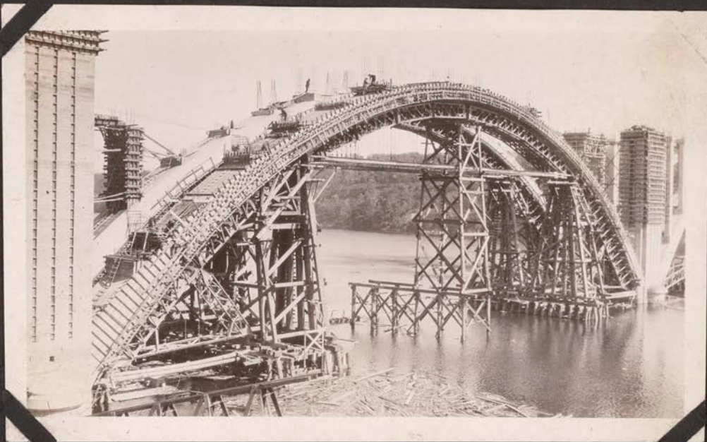
South Elev. Span 9 Ribs poured except Key Sections. Oct. 1 1926
