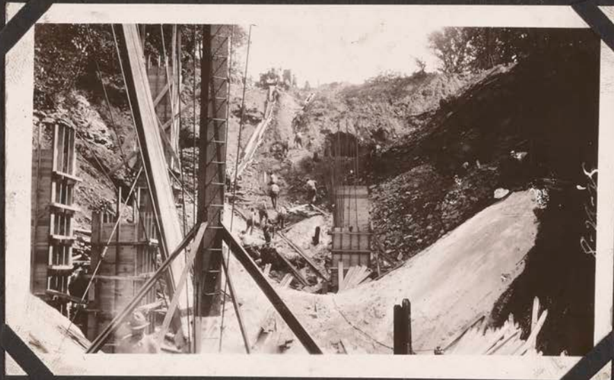
East Approach, Aug. 28, 1925. Excavating and Pouring Column Footings.
