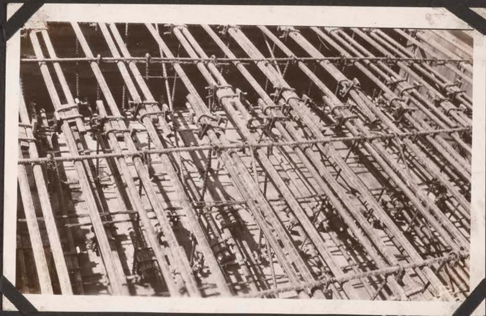
Typical Splice in Arch Rib Reinforcing.
