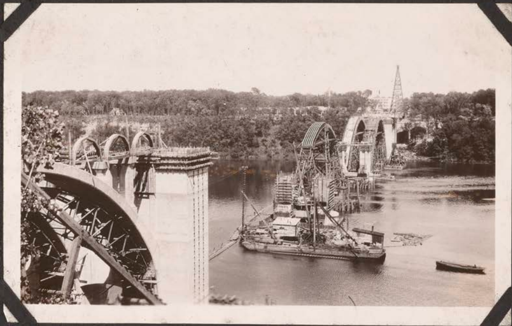
Progress View Looking East July 10, 1926.
