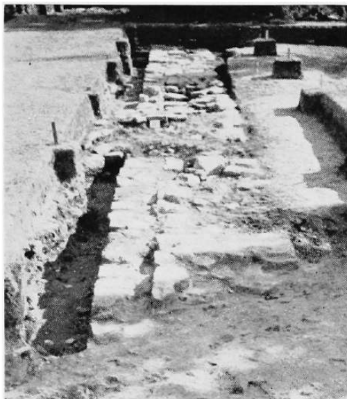
FOUNDATIONS of the outer wall
