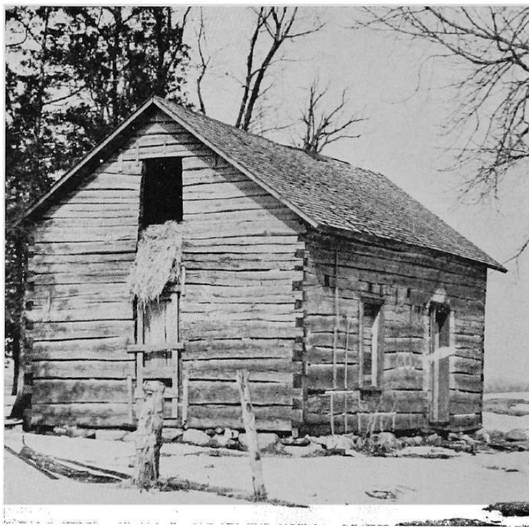
THIS log house near East Union in Carver County, photographed by the author in 1939, was the first cabin to interest him. It was built with dovetail corners by Scandinavian settlers.
