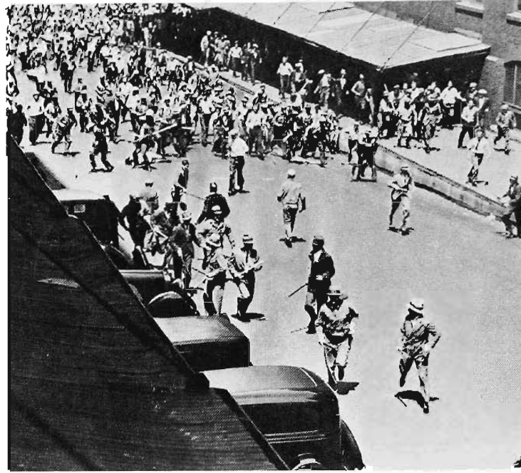
CLASS HATRED boiled to the surface in the old market area as strikers routed the citizens' army on May 21 in what truckers later took to calling the "Battle of Deputies Run."
