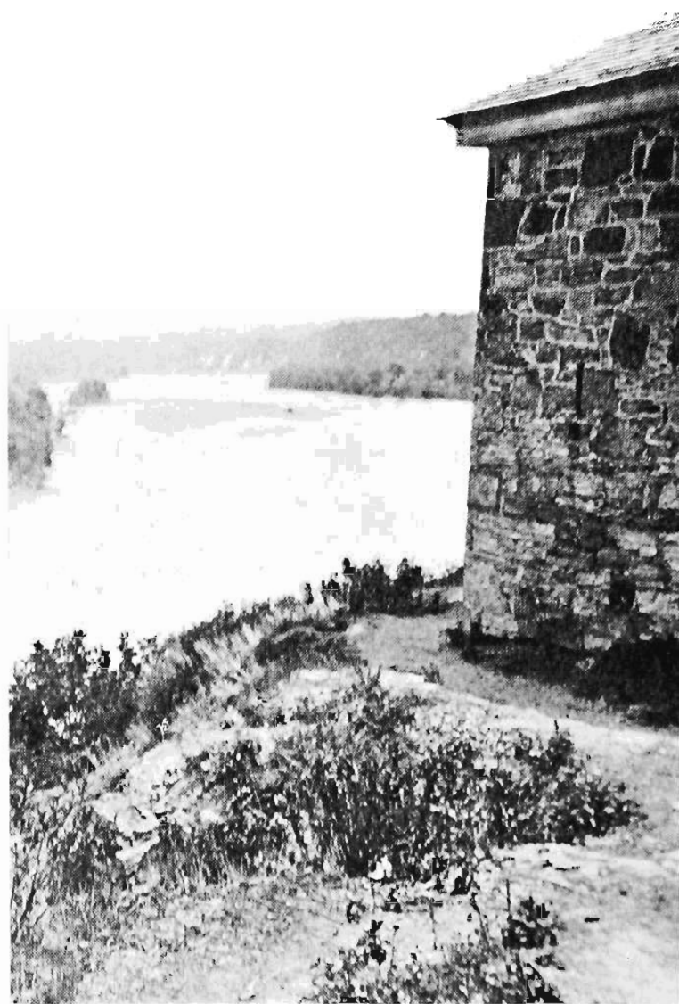
THIS NINETEENTH CENTURY scenic panorama, perhaps only incidentally including a close-up of the Pentagonal Tower, provided otherwise unknown information about roof pitch and placement of gun slits.
