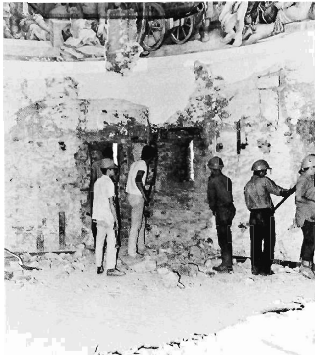
INSIDE THE ROUND TOWER crews chipped off the plaster (including, unavoidably, the Richard Haines mural) and opened the long-blocked gun slits as a prelude to the actual restoration.
