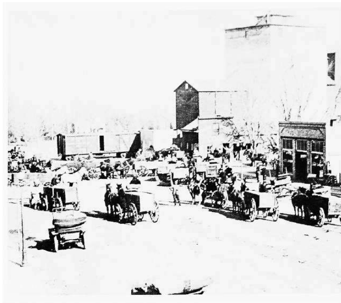
IN THE early twentieth century, railroads and grain elevators maintained commanding positions, economically and architecturally, in Minnesota communities.
