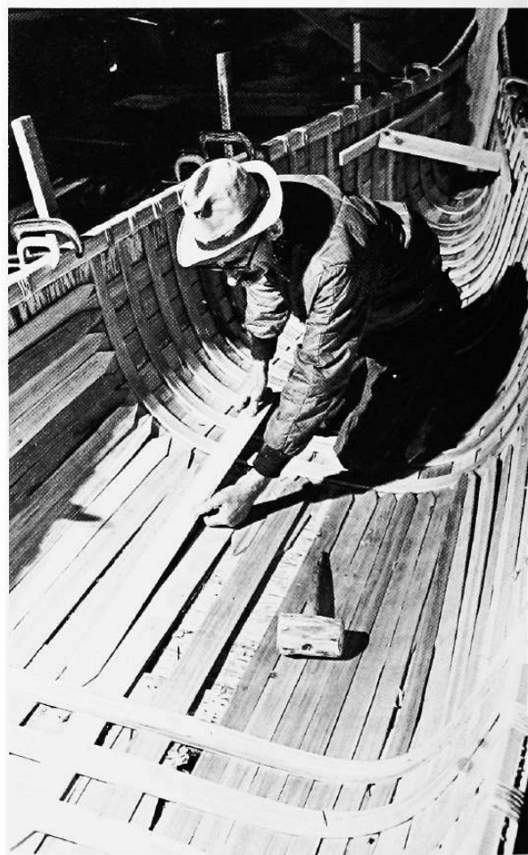
PLANKING IS INSERTED and pounded in under the ribs. The ends of the ribs are caught under the gunwales, thus applying pressure against the planking which in turn exerts pressure against the bark and maintains the form of the canoe.
