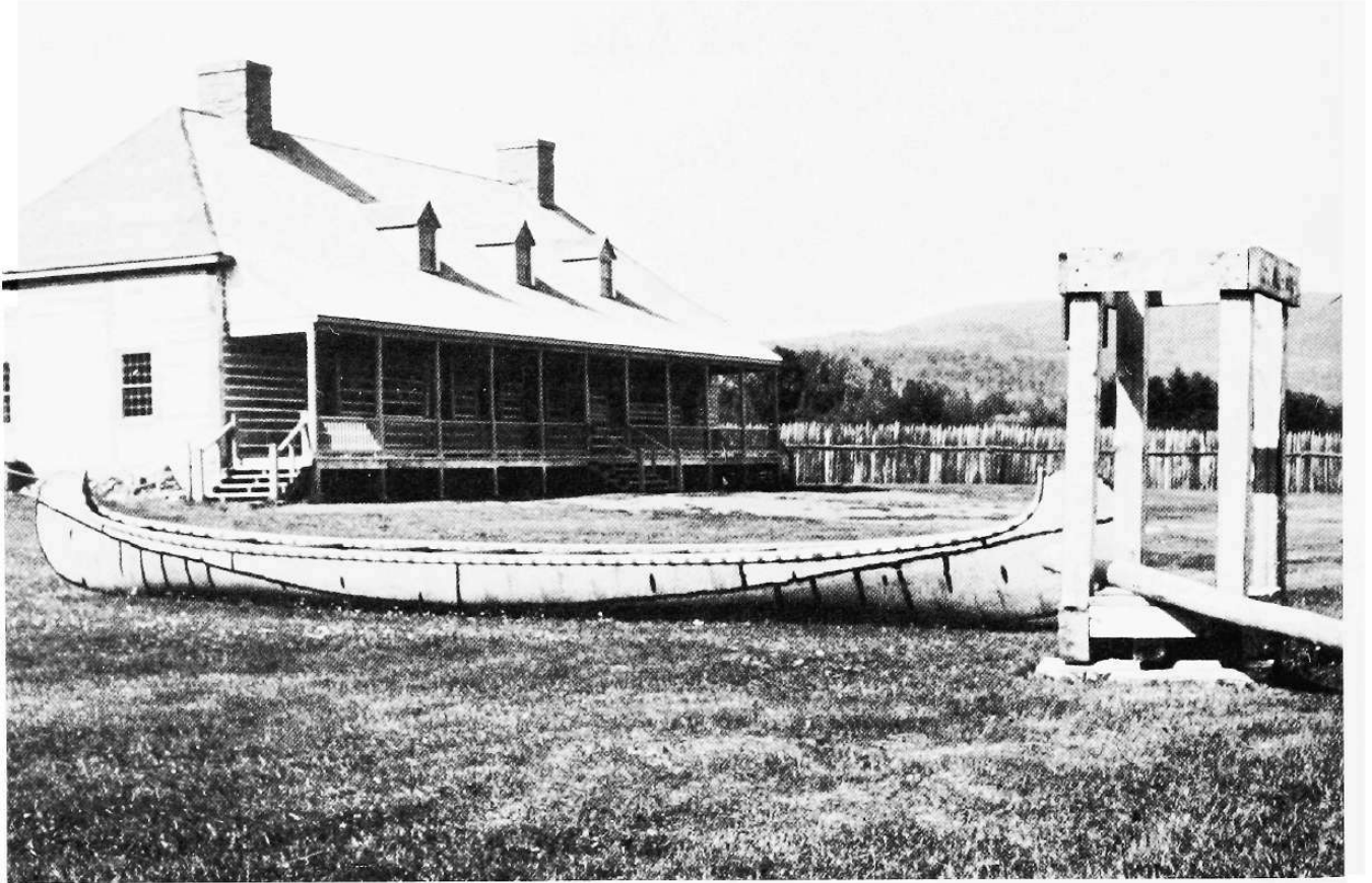
THE GREAT HALL is the only building completed thus far in the reconstruction of Grand Portage. A replica of a 34-foot Montreal canoe and one of a fur press are in the foreground.
