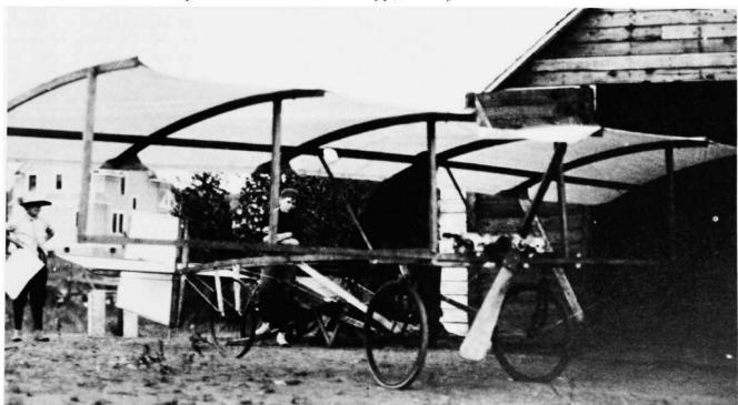
wing on Parker's machine had a span of 23½ feet and a width of 6½ feet, the exact dimension of the Farman wing. In mid-August this machine was smashed when Parker attempted to fly it. It was probably underpowered and did not get far off the ground.
