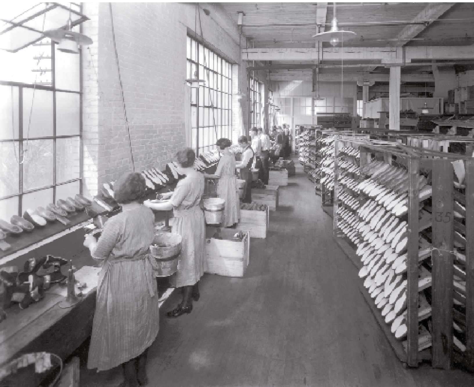
Piecework employees in the shaping department of Minneapolis's Robertson Shoe Company, 1621 Hennepin Avenue, 1922
