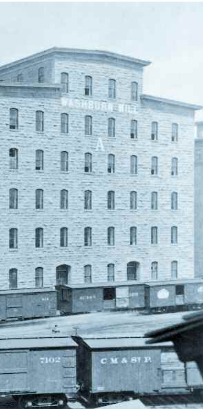
Rail service to the rebuilt Washburn A Mill on the Mississippi's west bank, about 1882
