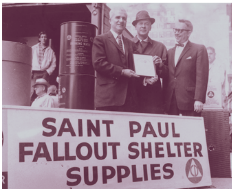
Stocking a civil defense shelter in St. Paul’s First National Bank, 1963
