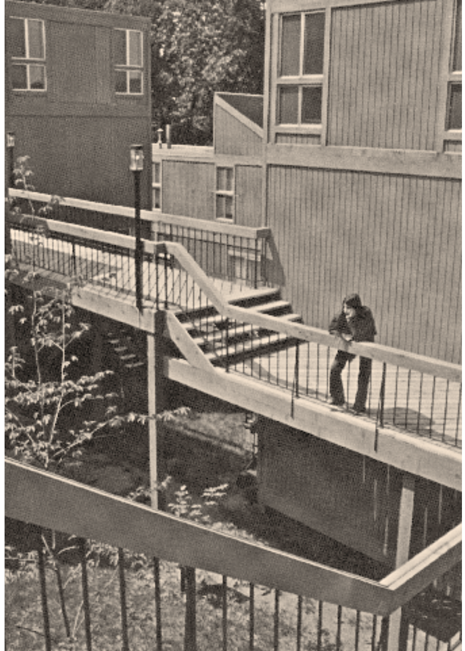
Design innovation: Tree-loft apartments connected by an elevated boardwalk; photo in special issue of Northwestern Bell Magazine devoted to livable communities, 1972.
