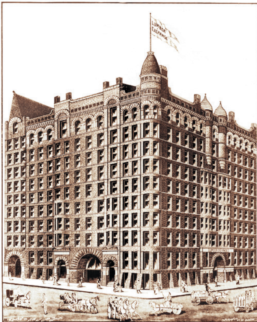
Early design for enlarging the Lumber Exchange. The addition (left side) along Hennepin Avenue is ten stories, like the original section, and preserves the original roofline.
