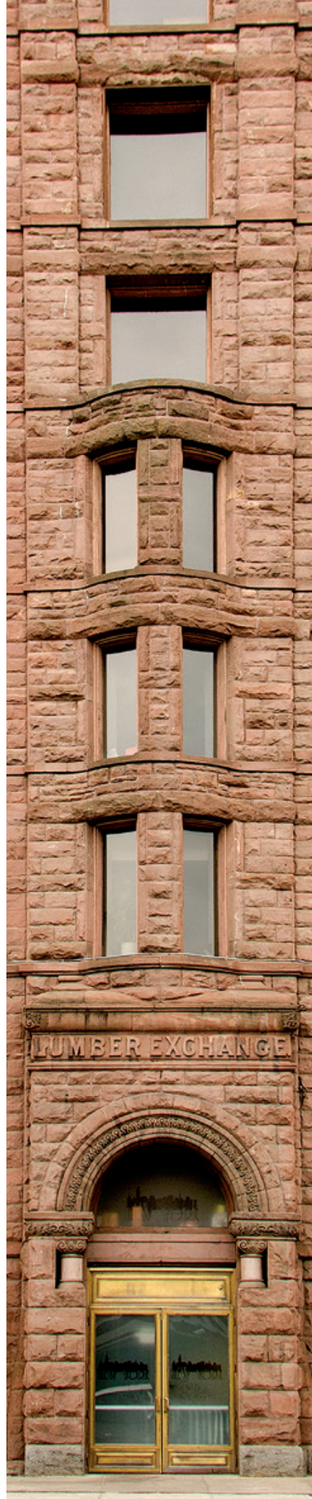
Detail of the Lumber Exchange’s rock-faced façade, 2014. This section was the terminus of the original building’s Hennepin Avenue side.
