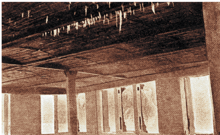
Tenth-floor ceiling in the original section after the fire, showing uninjured fireproof arches; Inland Architect, August 1891, page 9.
