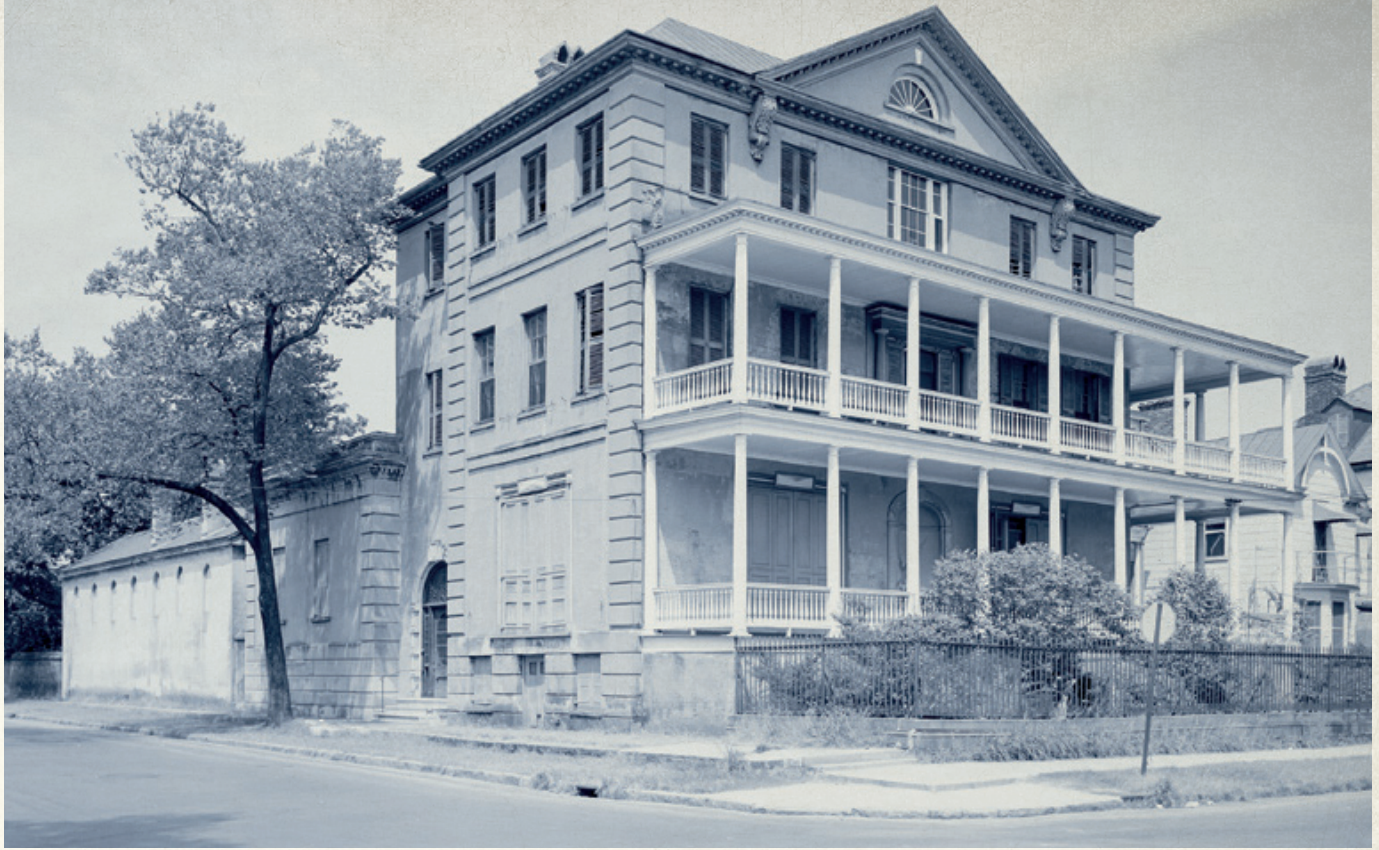
The Charleston, South Carolina, house of William Aiken, 1963 view.
