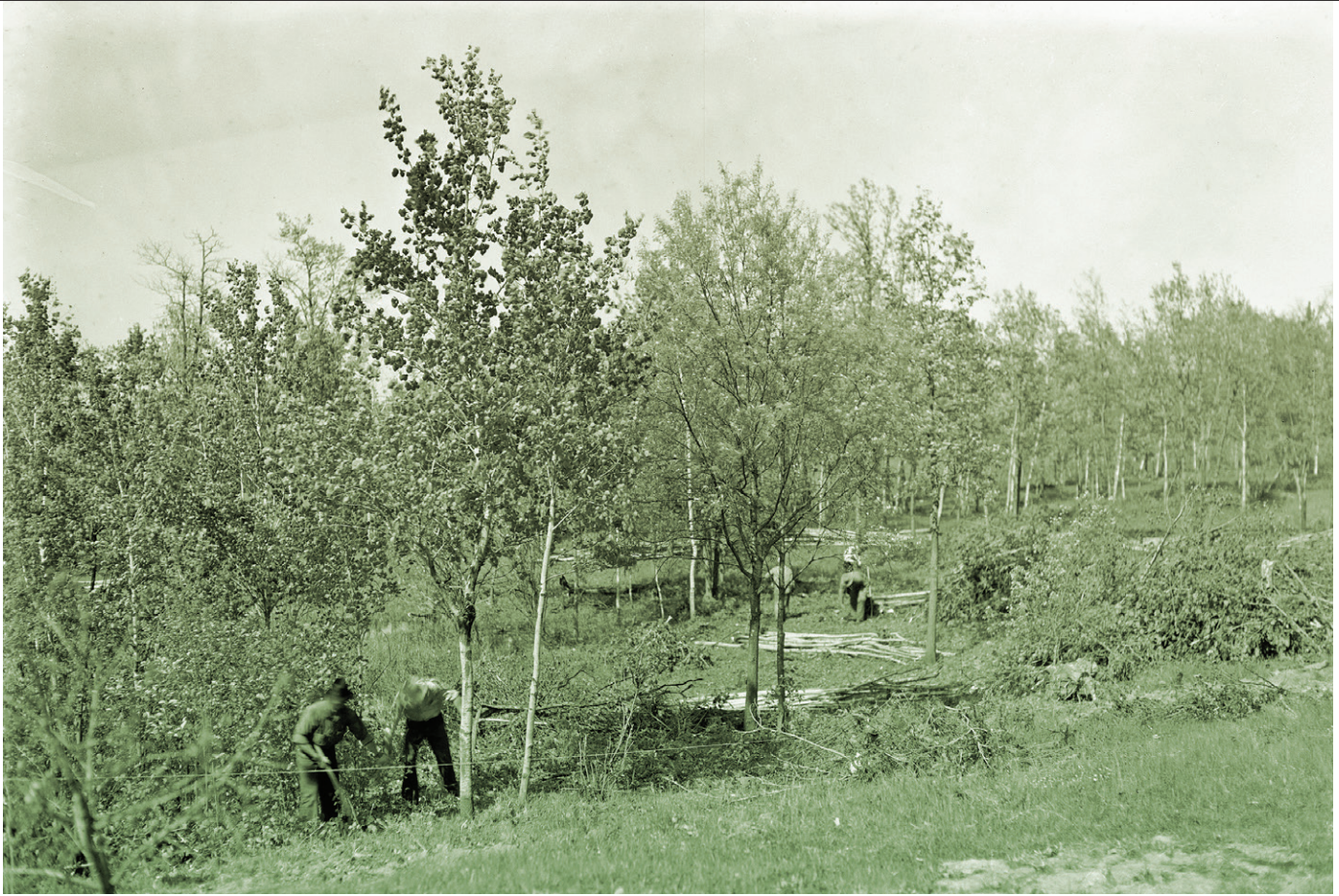
WPA work on Pierz course, May 25, 1936. The tiny town was the first in the state to have its proposal for a golf course approved by the WPA.
