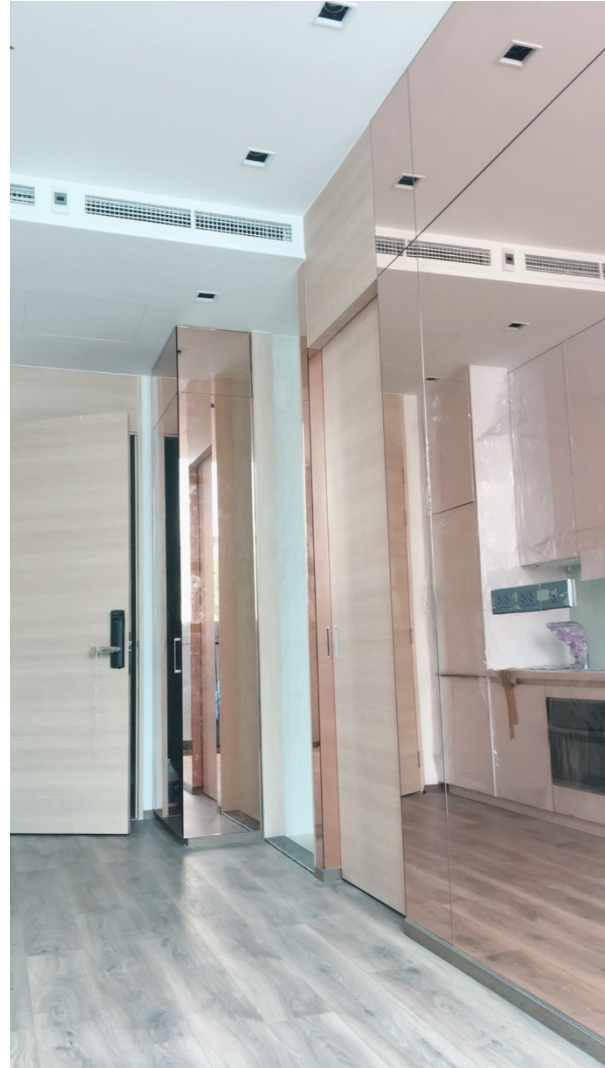
Sales Gallery Progress : Mock Up Room 'A'
