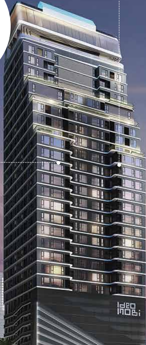
SOLAR CELL PANEL EVERY UNITS
