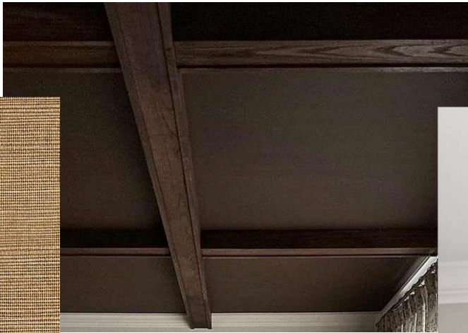
DARK STAINED BEAMS ON CEILING
