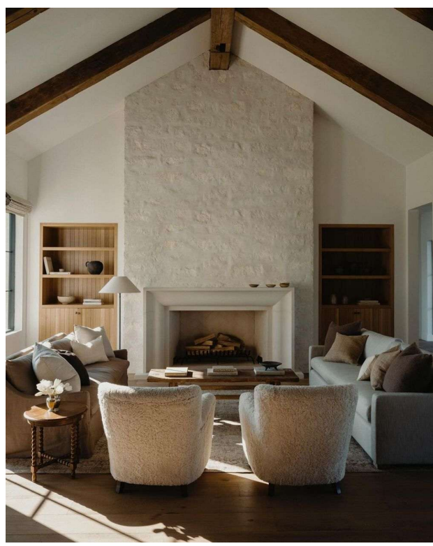
STAINED BEAMS ON CEILING, SIMILAR STYLE
