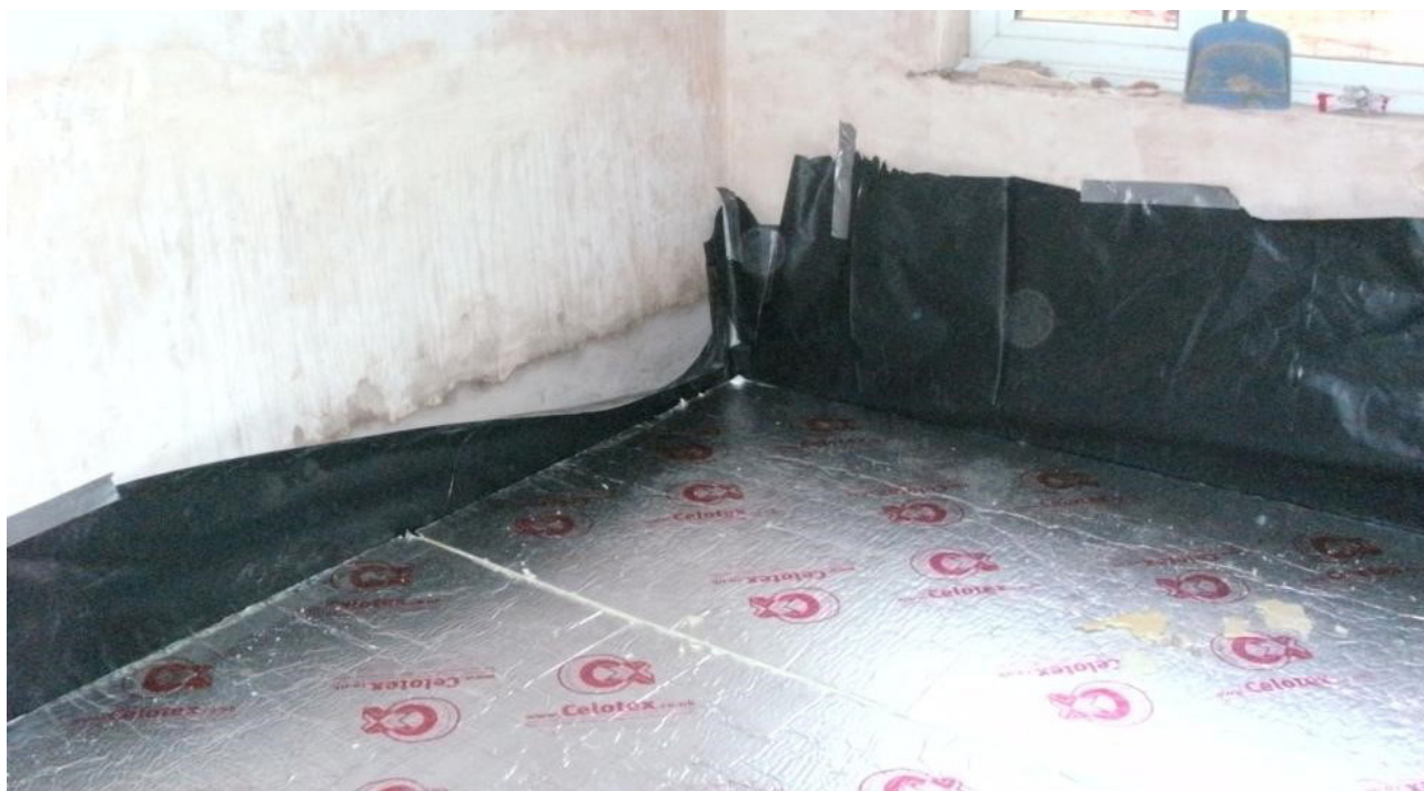
Figure 18 Damp Proof Membrane as air barrier, to be taped up internal walls and joined to plaster layer behind skirting
