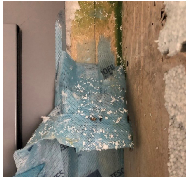
Figure 14 Photo of airtight tape that has been applied to an unprepared surface
