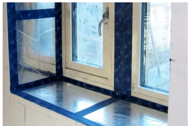
Figure 15 Airtightness tape applied to a window reveal that closely follows the contours of the reveal
