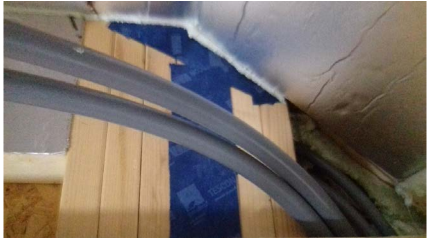
Figure 30 Multiple timber posts penetration roof air barrier
