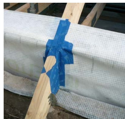
Figure 21 Photo of airtight membrane connecting internal air barrier to membrane over the roof joists
