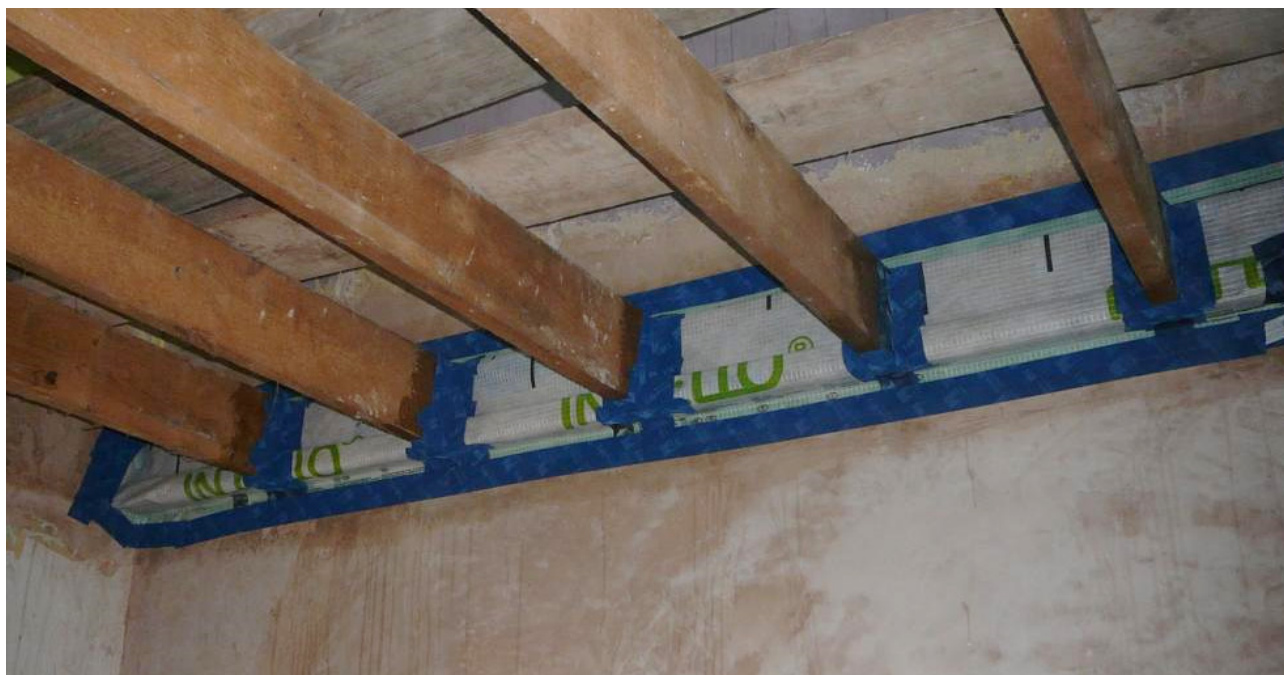
Figure 24 Intermediate floor to wall junction. Air barrier is wet plaster with membrane and airtightness tape around the joists.
