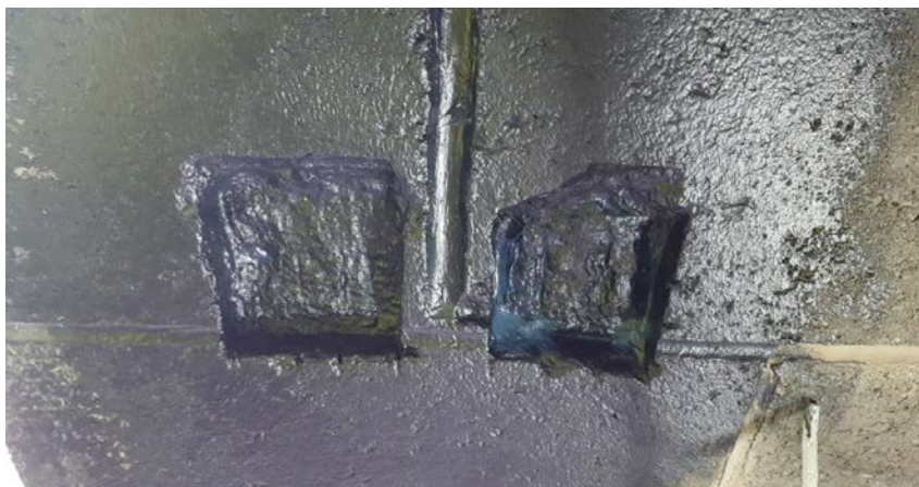
Figure 16 Chasing in blockwork for electrical switches and wiring, treated with an airtight paint that paints on blue and dries black when airtight
