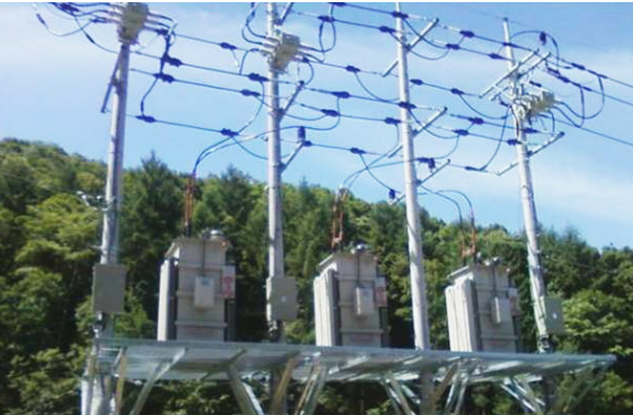
Picture of Installation Case (PVR 7000KVA)
