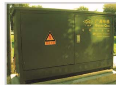
户外电缆分接箱 Outdoor cable branch box
