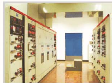
低压开关柜GCK GCK low-voltage withdrawable switchgear
