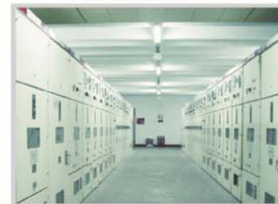
高压开关柜XGN XGN high-voltage switch cabinet
