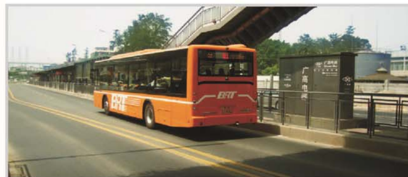
广州BRT建设工程美式箱变 Operating in BRT construction project American-type box transformer substation
