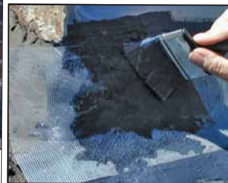
For added strength and flexibility, a fiberglass fabric is embedded between 2 coats of FlashSeal Elastomeric Sealant
