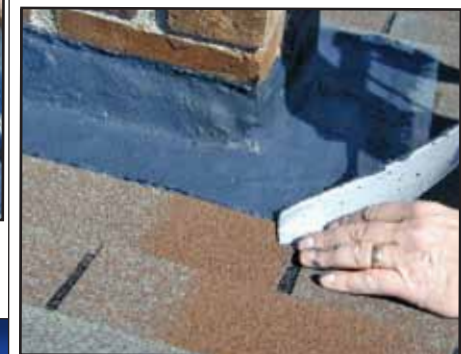
In most cases the roof deck and chimney are taped off to produce a neat appearance of the finished application
