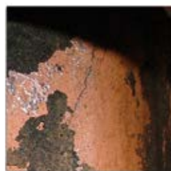
This crack may be small, but it could open as wide as 1/4 inch when the flue is overheated.
