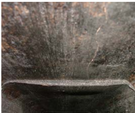
A crack like this can allow deadly gases to leak into the home, and can open the way for a chimney fire to turn into a house fire
