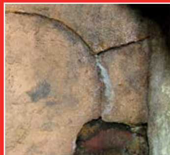
Damaged flue: Notice the moisture and the missing piece of flue tile.
