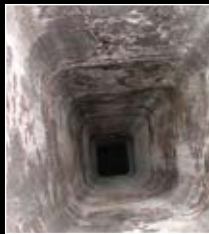
Cracked flue tile
