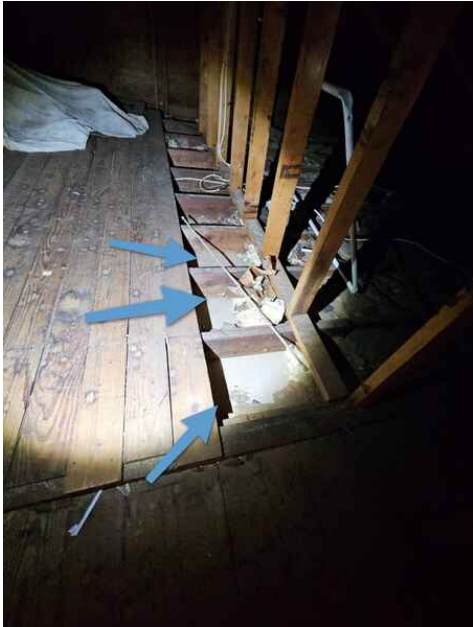
Missing insulation throughout
