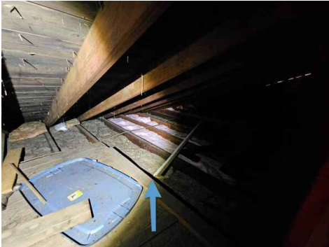
Insufficient insulation throughout the attic
