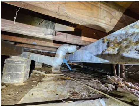
Duct not to be sealed by duct tape
