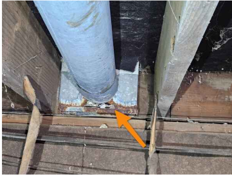
Rusted out and has a hole
