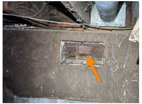
Damaged vent cover
