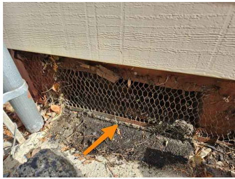
Improper vent cover
