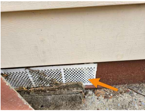
Improper vent cover
