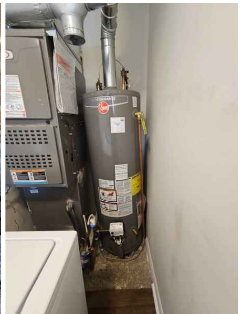
Water heater is leaning due to damaged subflooring
