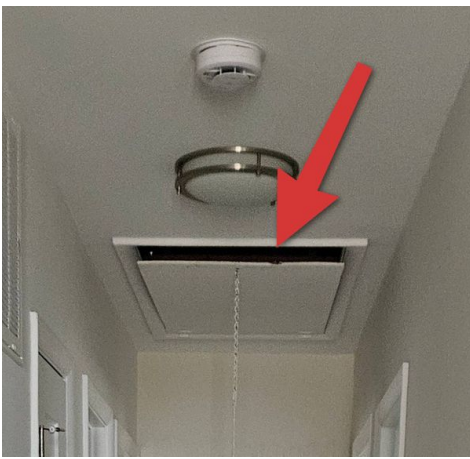
Access door does not stay shut nor latch shut
