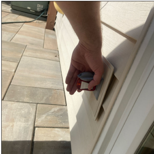
Patio receptacle not GFCI, reverse polarity
