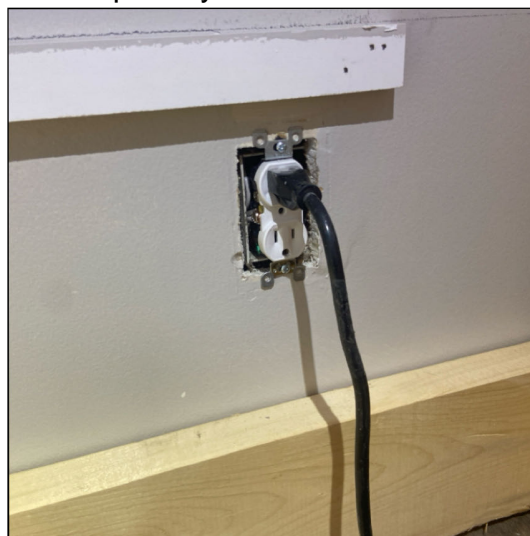
Sump pump receptacle
