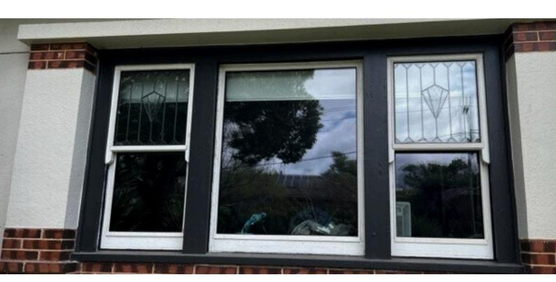
For heritage windows with sash designs, the use of acrylic becomes problematic, making it nearly impossible to employ secondary glazing successfully. These factors, combined with the impact secondary glazing has on the aesthetic appeal of windows, make it an unsuitable choice for soundproofing historic period windows.
