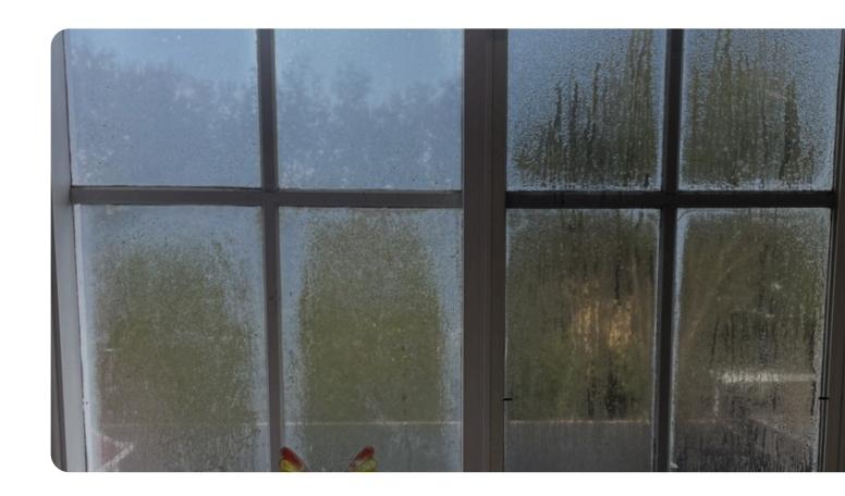
The primary issue arises with the polysulphide secondary seal around the IGU. Some companies encase the double glazing in a square-cut rebate, filling it with silicone. However, this approach poses two critical problems: most silicones are incompatible with the polysulphide seal, and if there's a gap in the rebate seal, water infiltrates, becoming concentrated saturated water vapour that corrodes the polysulphide seal, resulting in double glazing failure.
